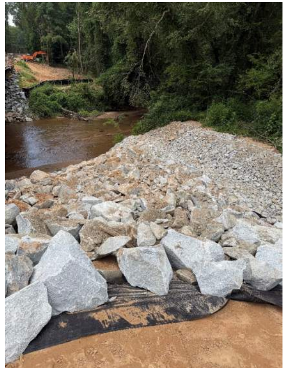
Rip Rap being installed on sides
