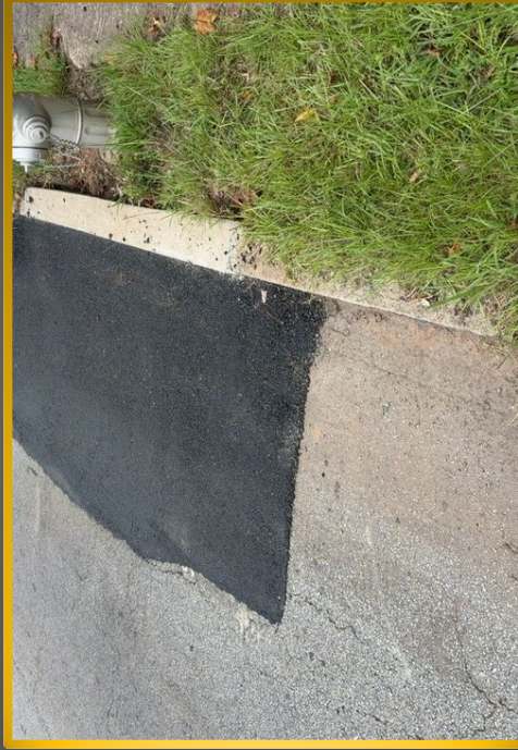
Fire hydrant leak- Road cut to stop the leak and restoration
