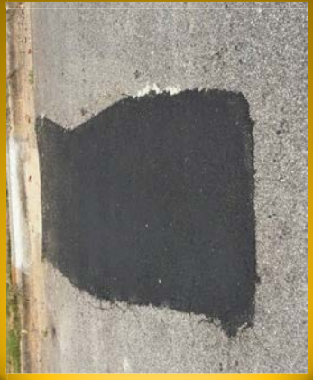
Water meter repairs road cuts and restorations
