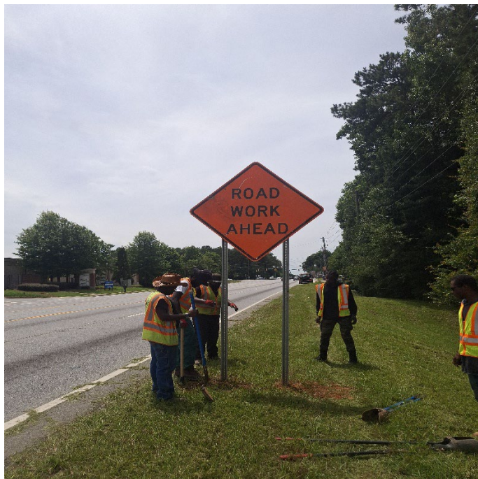
TCCD – Advance WARNING Signs Installed
