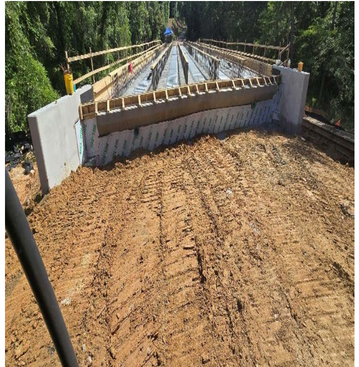
South side dirt grade prior to steel tying
