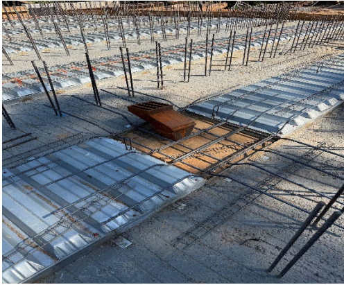
Top of Drain installed
