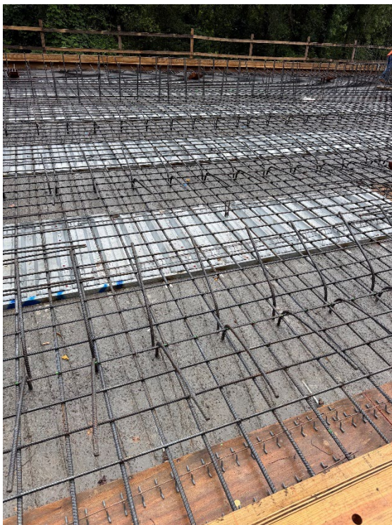
Rebar bent and tied
