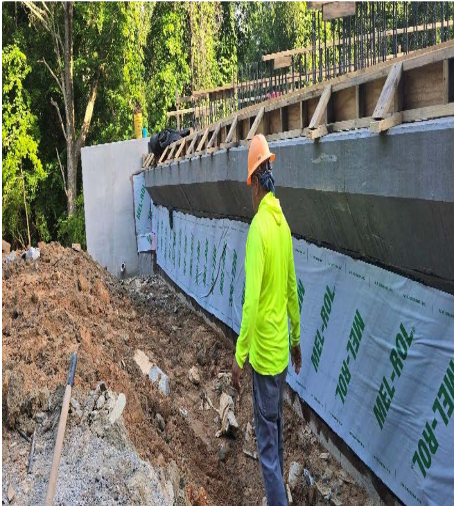
Waterproofed end walls at both bents
