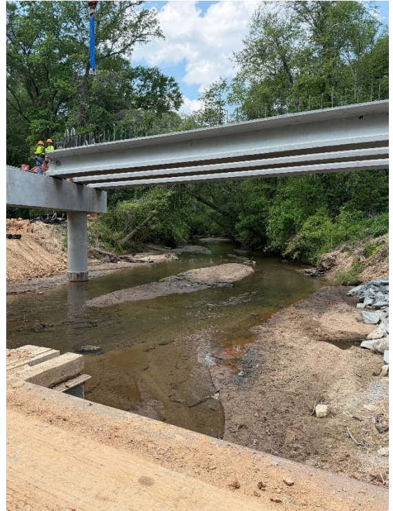
99' beams over creek
