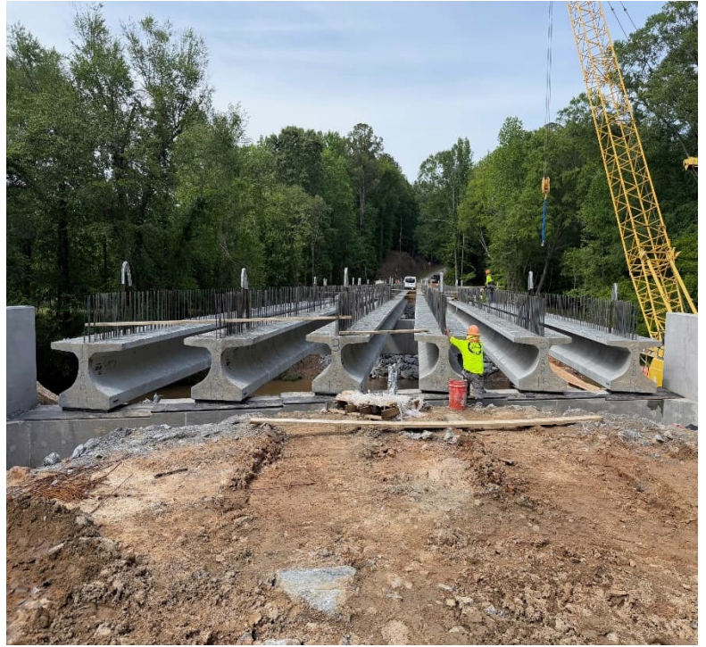
All beams installed
