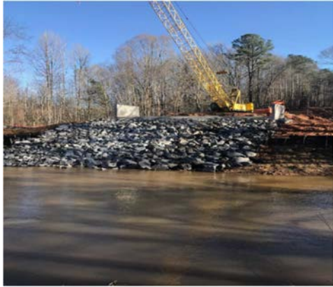
Rip Rap on slope of Bent 3
