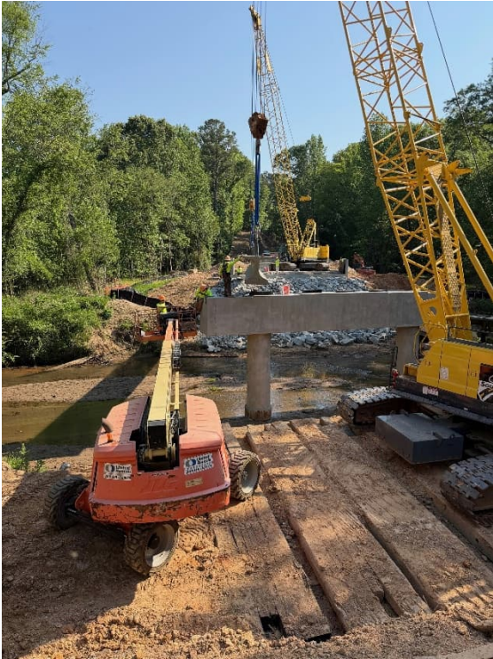
Setting 1 st beam (99' long)
