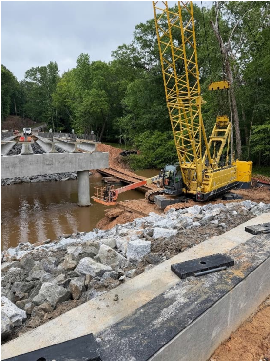
Span 1 Rip Rap installed
