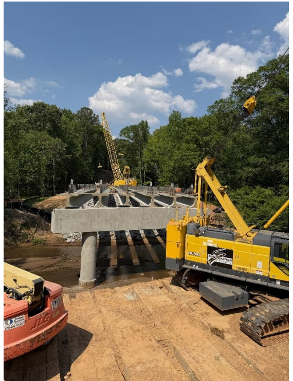
All 6 beams set for Span 2
