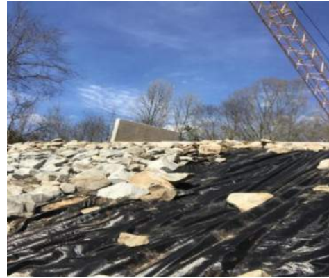
Fabric under Rip Rap
