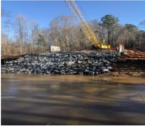
Rip Rap on slope of Bent 3
