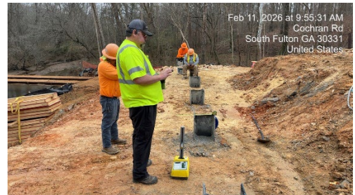
Bent 1 Piles driven
