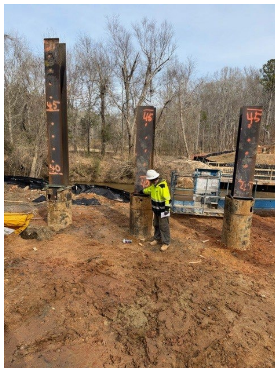
Validation of Piles driven on Bent 1
