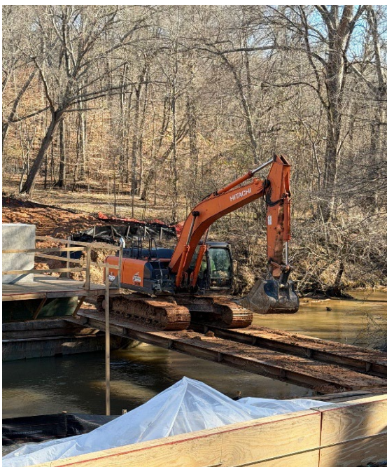
Using work bridge to move steel across
