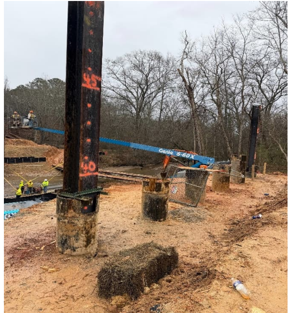
Test Piles in place Bent 3
