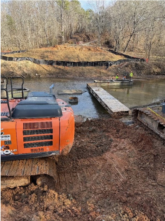
Relocated work bridge to save time
