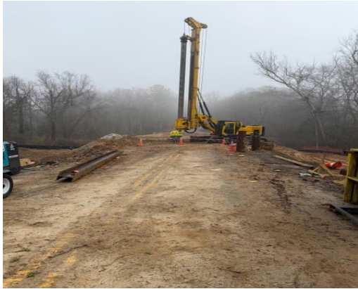
Maintenance of drilling Rig
