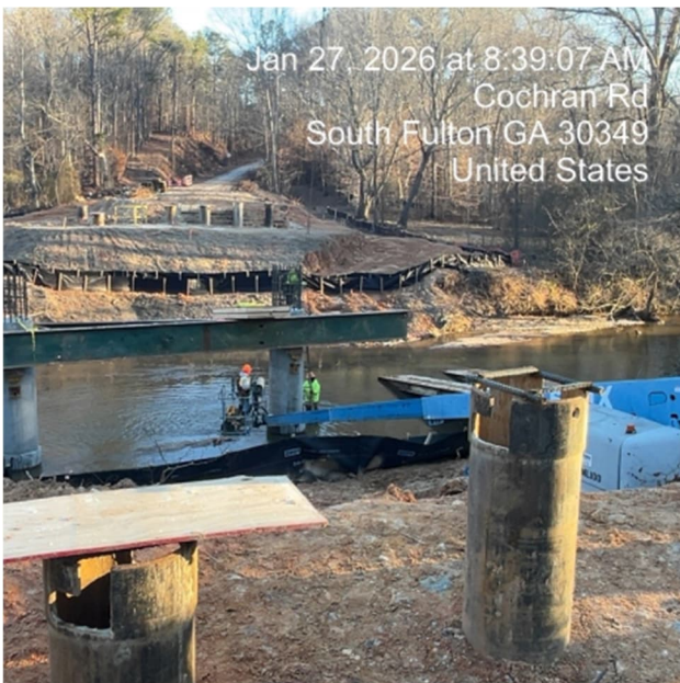
Forming Bent 2 Cap
