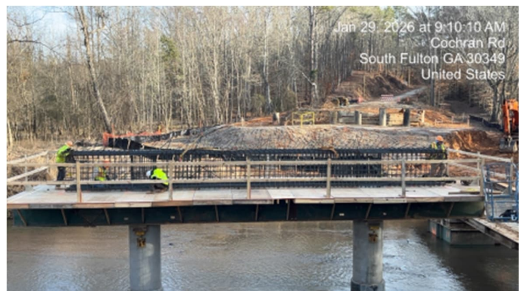
Steel rebar placement for Bent 2 Cap
