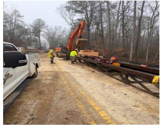
Preparing Hammer for pile driving
