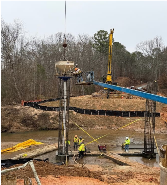
Pouring footer in Caisson 1
