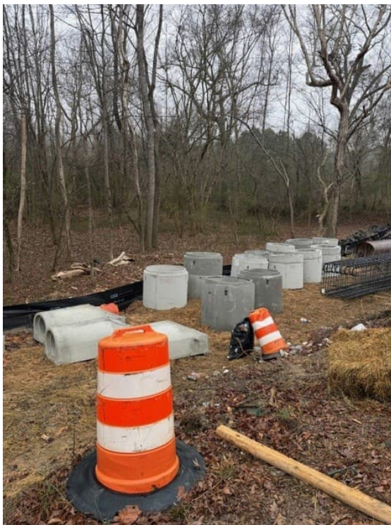
Foley Pipe Delivery
