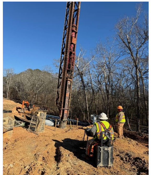
PDA Test Piles being driven
