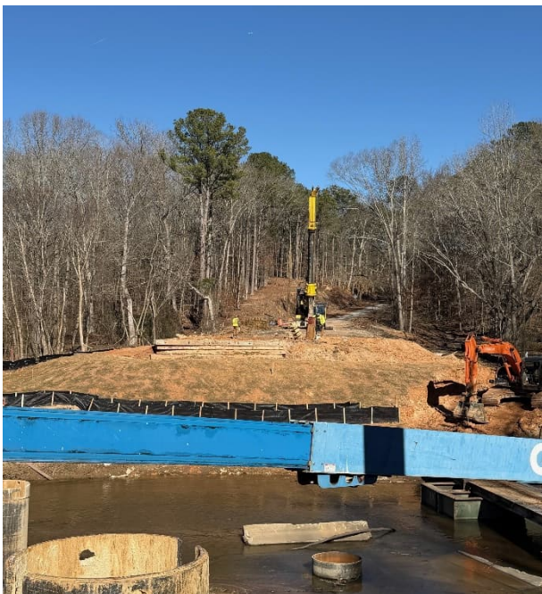
Drilling Pilot Holes on bent 3
