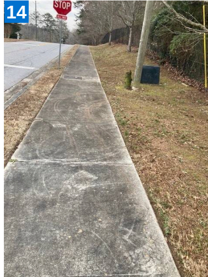
13 Piercing Rd. Before
