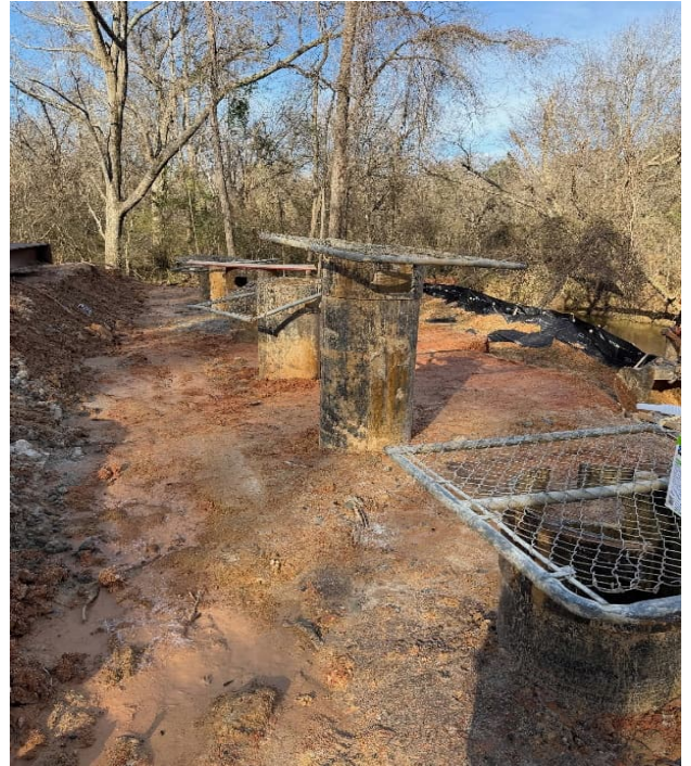
Bent 1 Pilot Holes drilled
