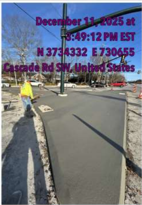
Large Median at Station 147+50
