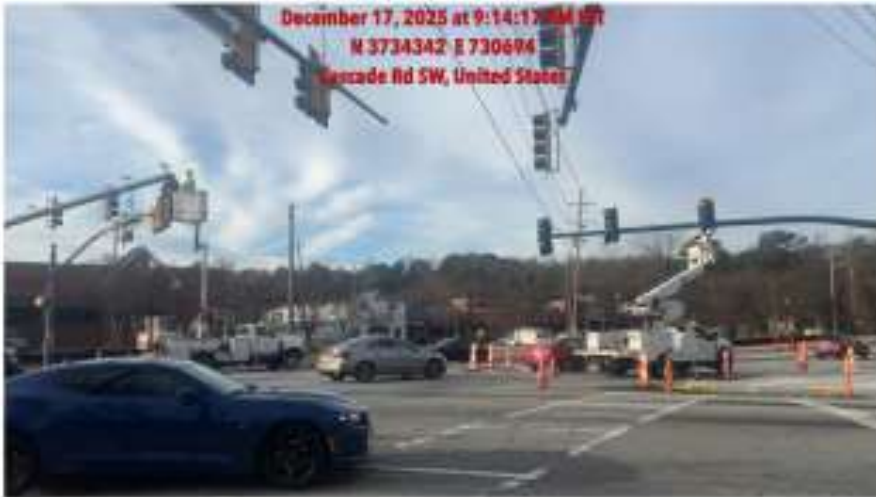
Reedwick working on new signal activation at Cascade and Fairburn Rd
