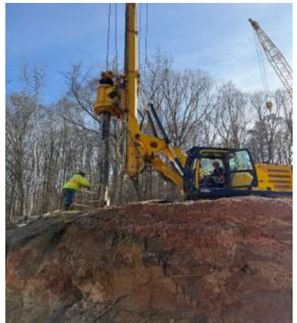
Drilling Pilot Holes on Bent 1
