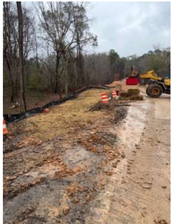
Erosion Control in place for rain 5 Dec 2025
