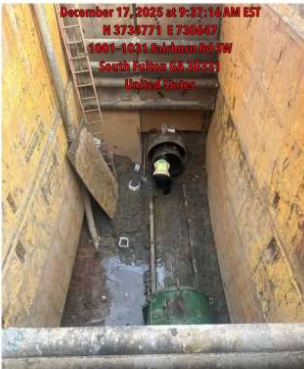
Pushing through 30 in pipe
