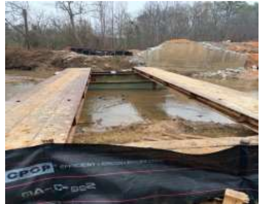
Work Bridge for drilling caissons
