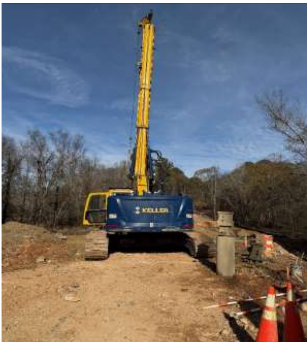
Drilling Pilot Holes
