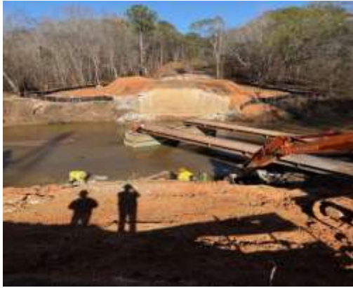
Work Bridge Installed 3 Dec 2025
