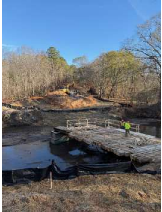
Demo Complete and Work Bridge complete
