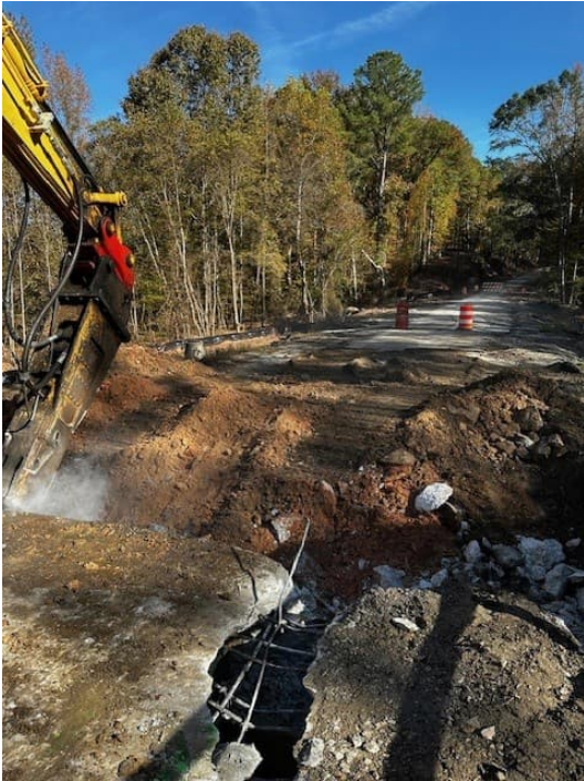
Bridge Demo 5 Nov 2025
