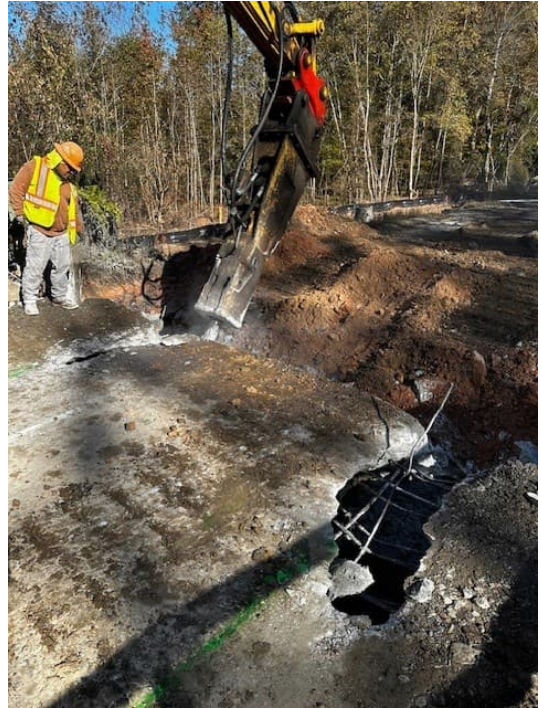
Bridge Demo 5 Nov 2025
