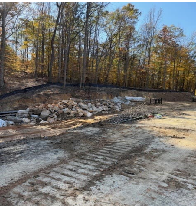
Crushing Rock and Separating Steel
