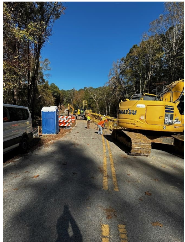
Setting up Crane 4 Nov 2025
