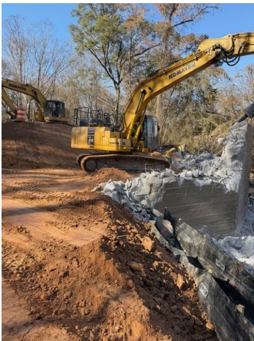
Bridge Demo 18 Nov 2025
