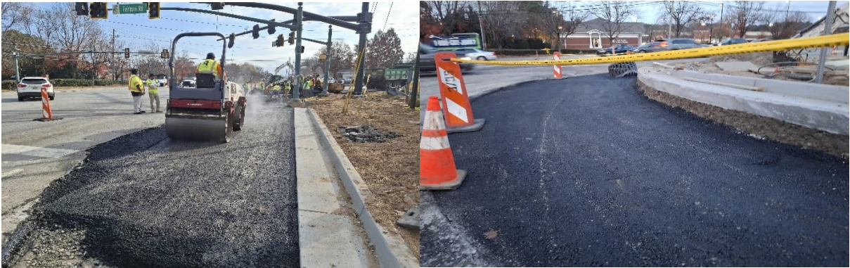
Asphalt Base Paving
