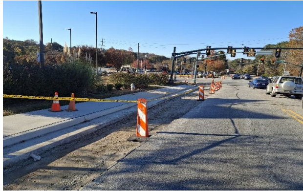
Grading Road Widening G.A.B
