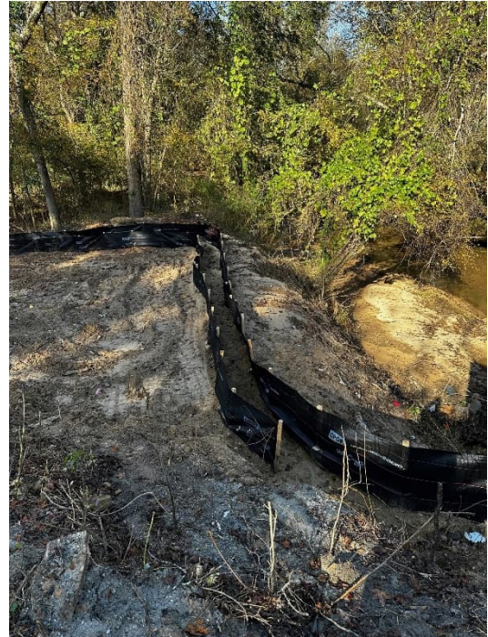
Double Row of Silt Fence in Place
