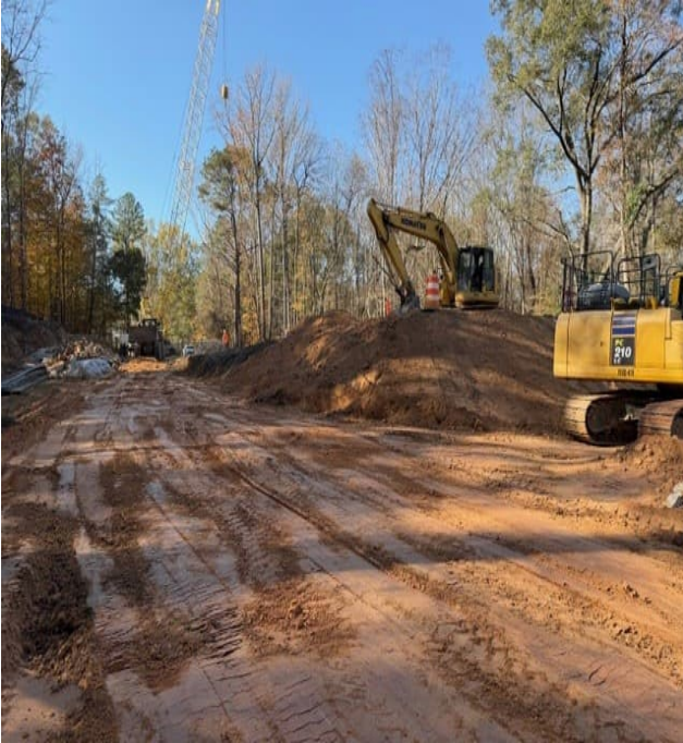
18 Nov Preparing for Work Bridge
