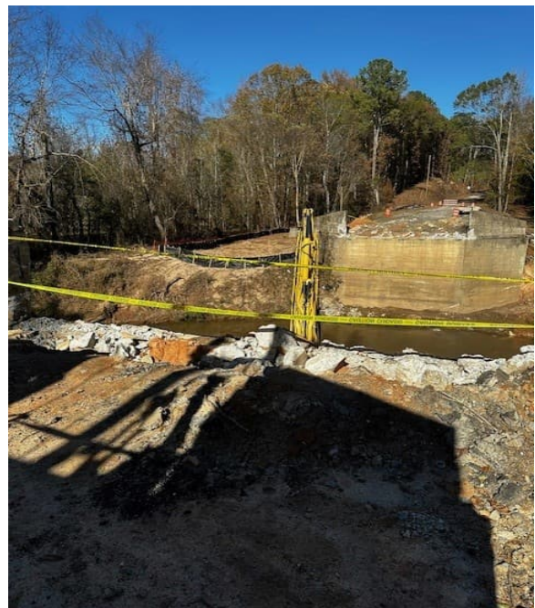
Bridge Demo 11 Nov 2025
