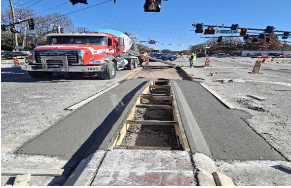
Median Curb and Widening Poured
