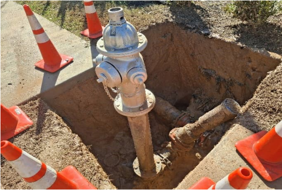
Fire Hydrant Relocate
