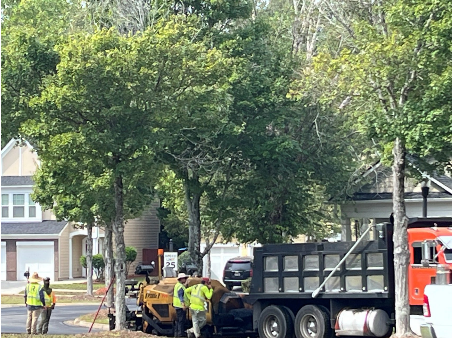
First Road Paved within The Lakes at Cedar Grove
