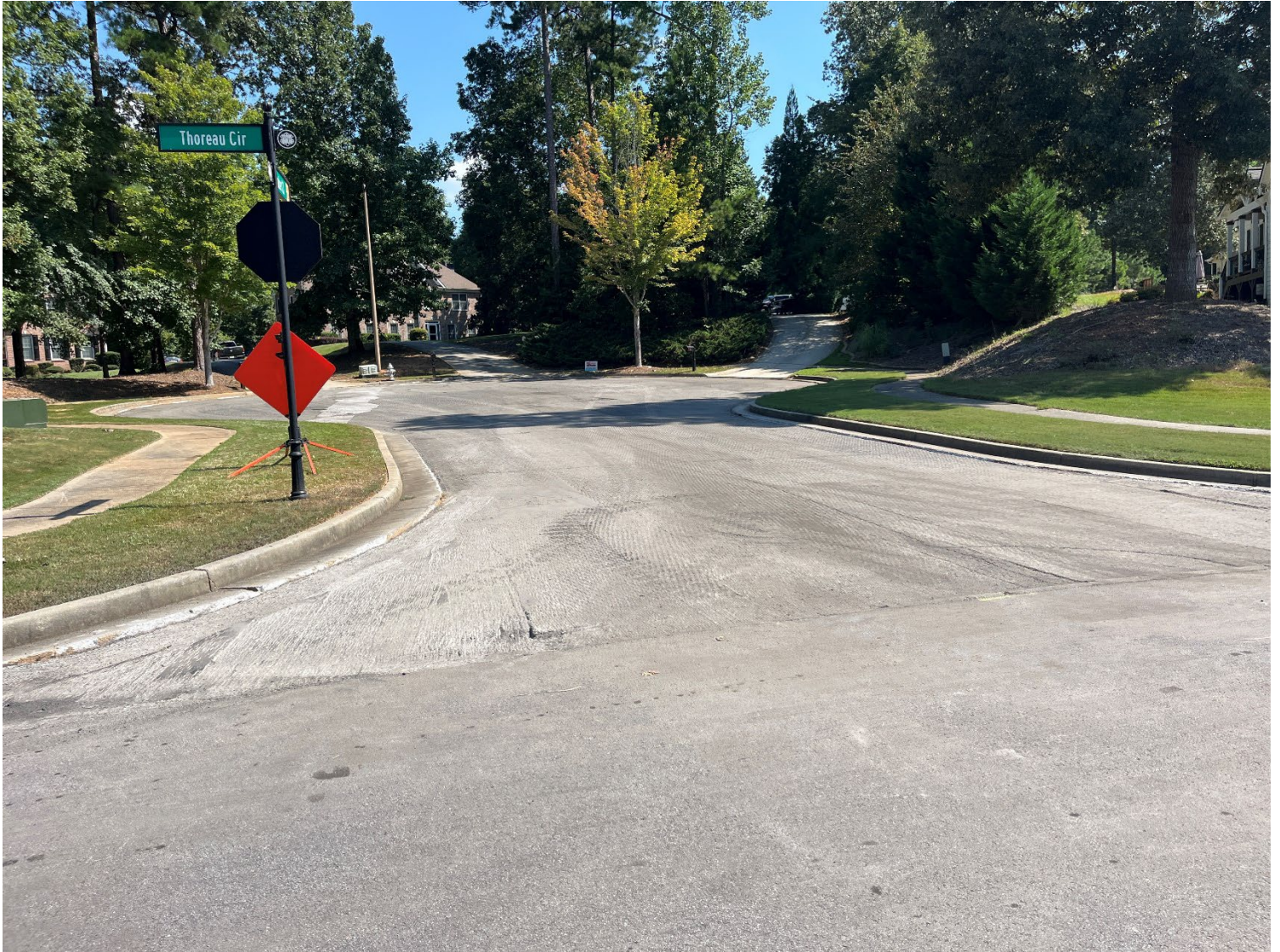
First Road Milled within Walden Park
