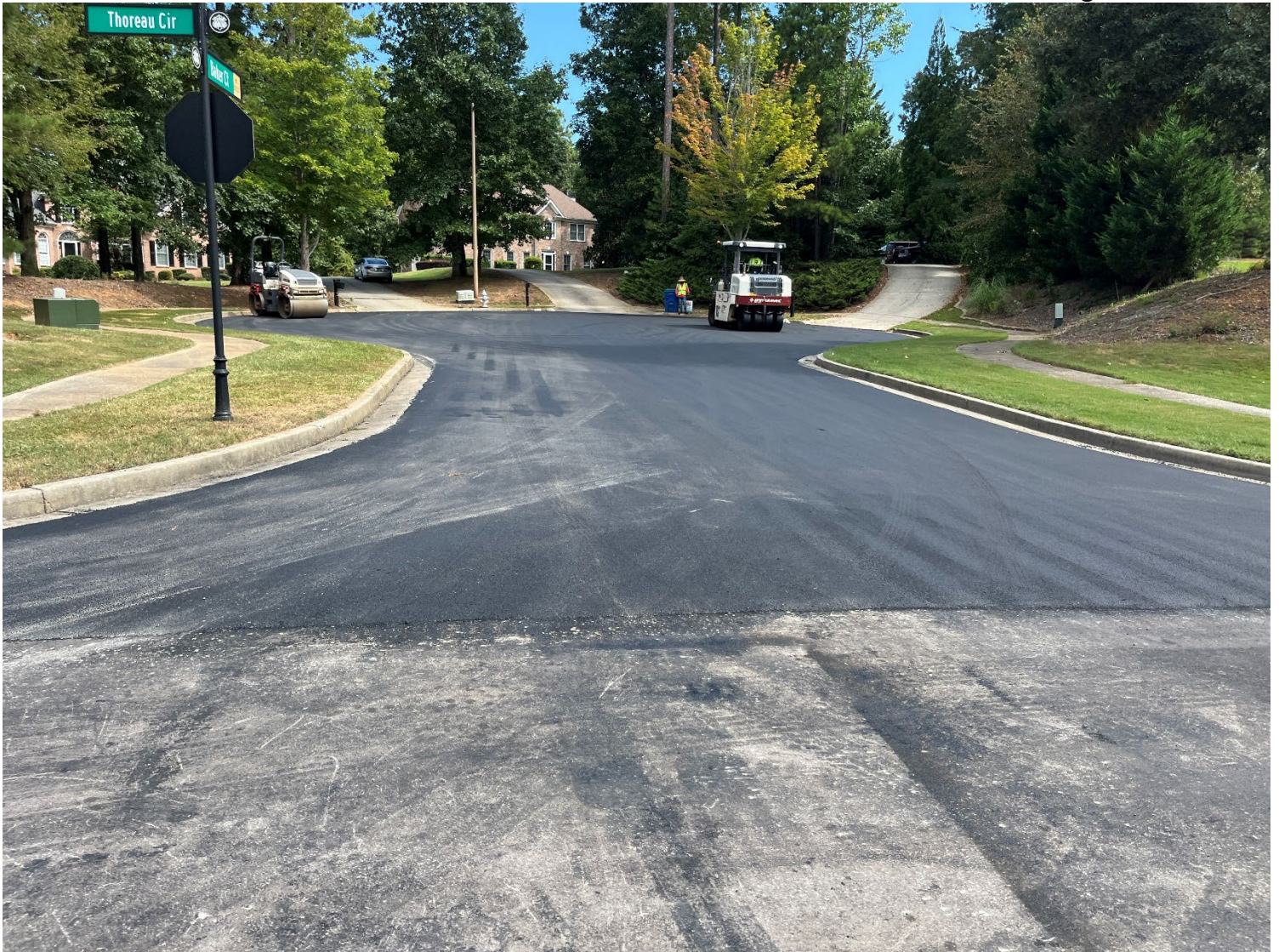
First Road Paved within Walden Park
