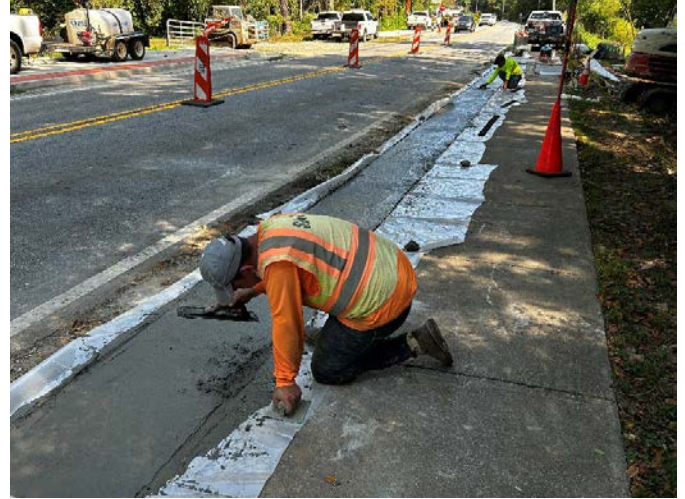
Catch Basin Ex-4
