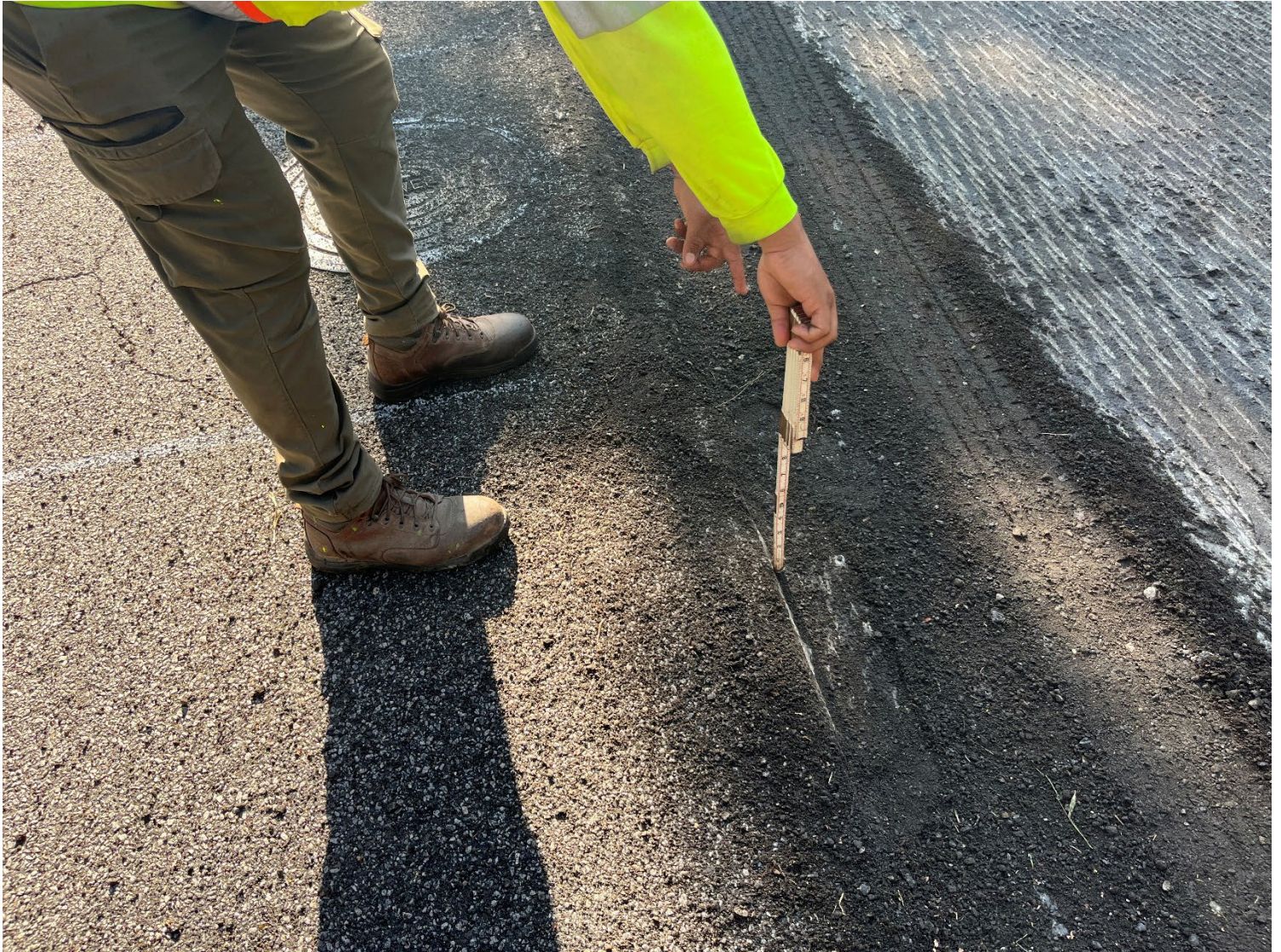
Measuring Milling Depth (1"1/2)
