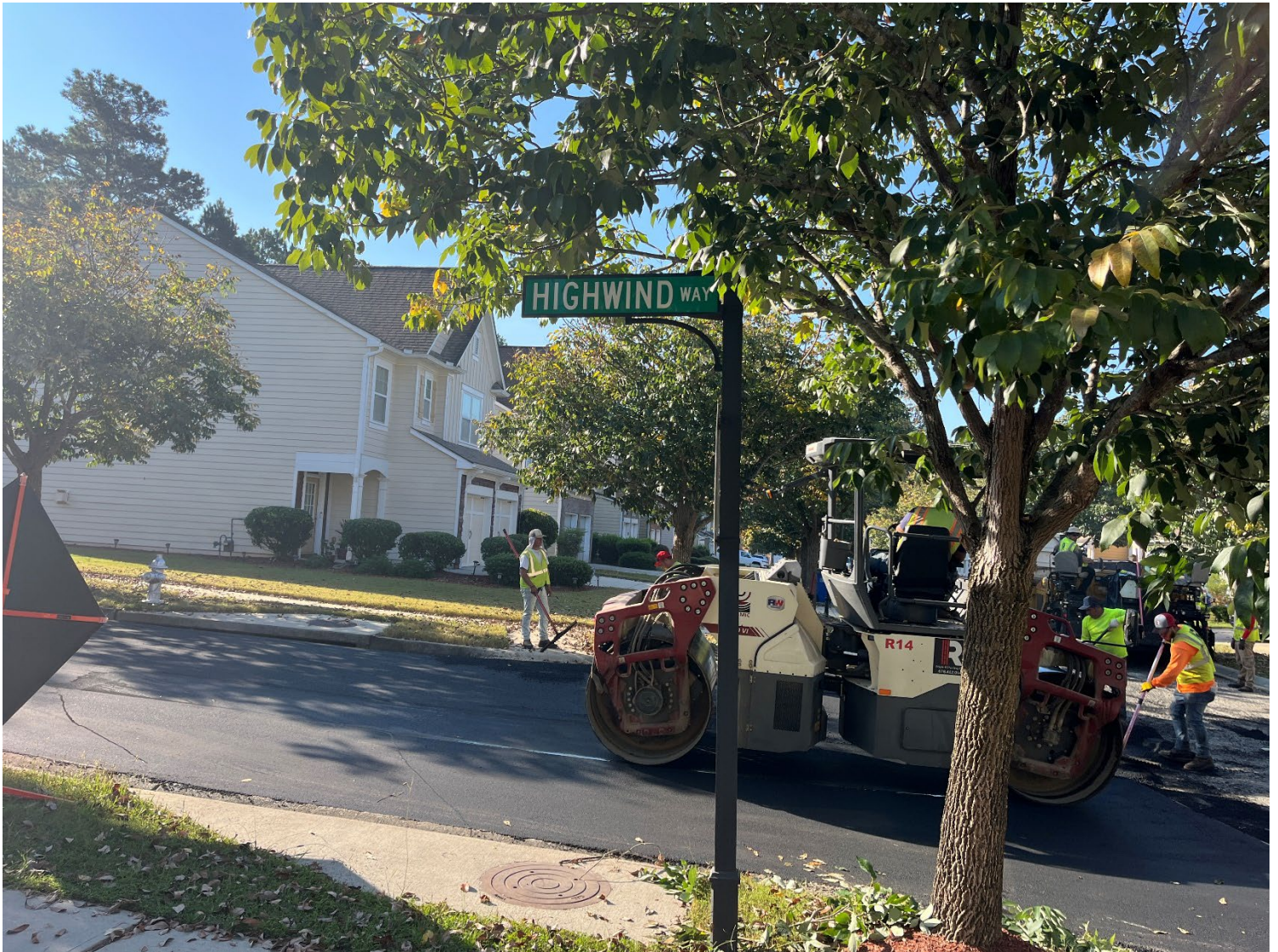
Paving Operation within The Lakes at Cedar Grove
