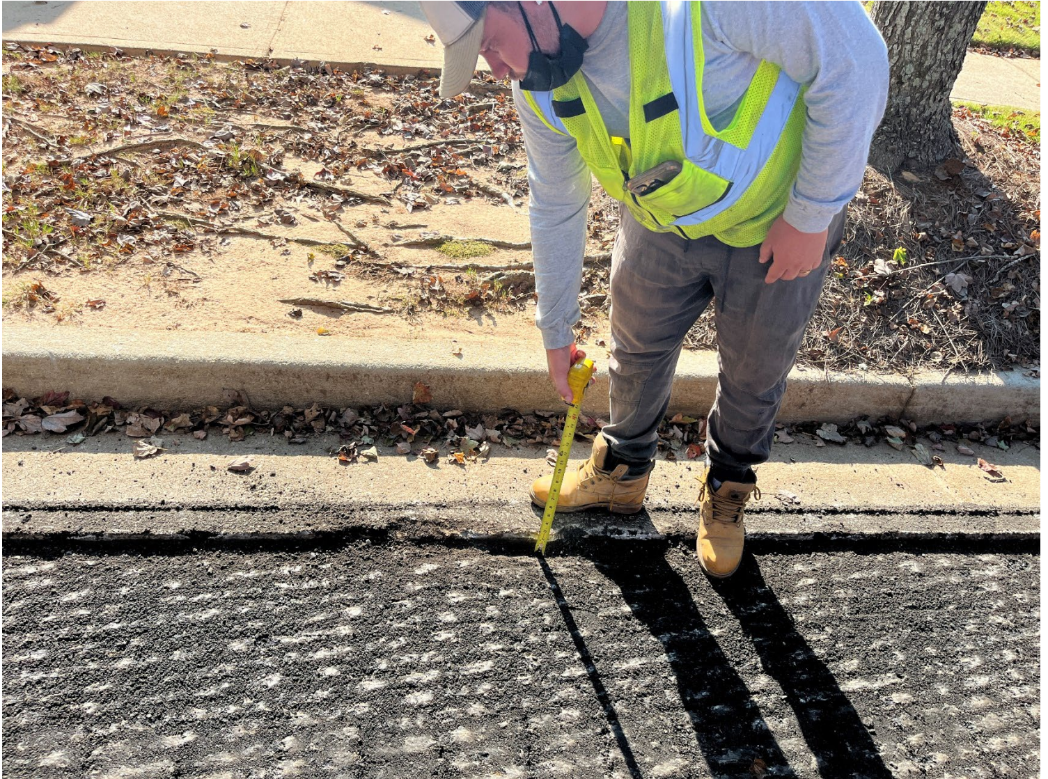
Measuring Milling Depth (1"1/2)
