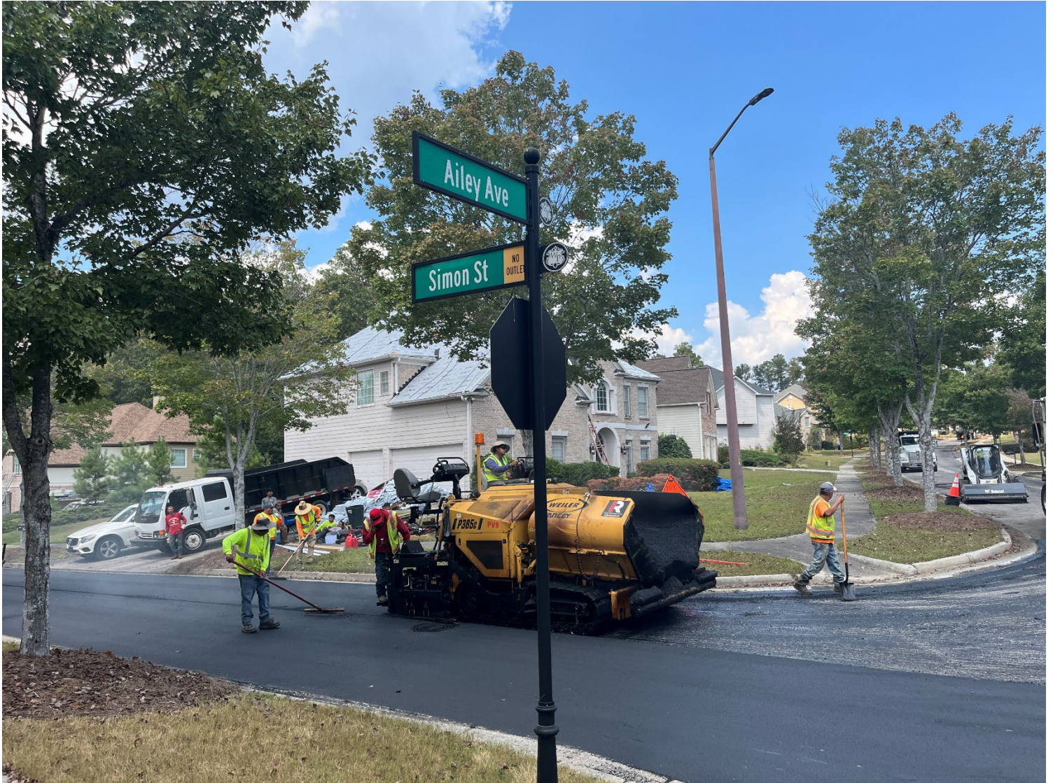
Paving Operation within Walden Park
