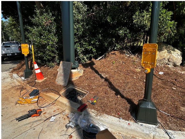
Pedestrian Meter Install
