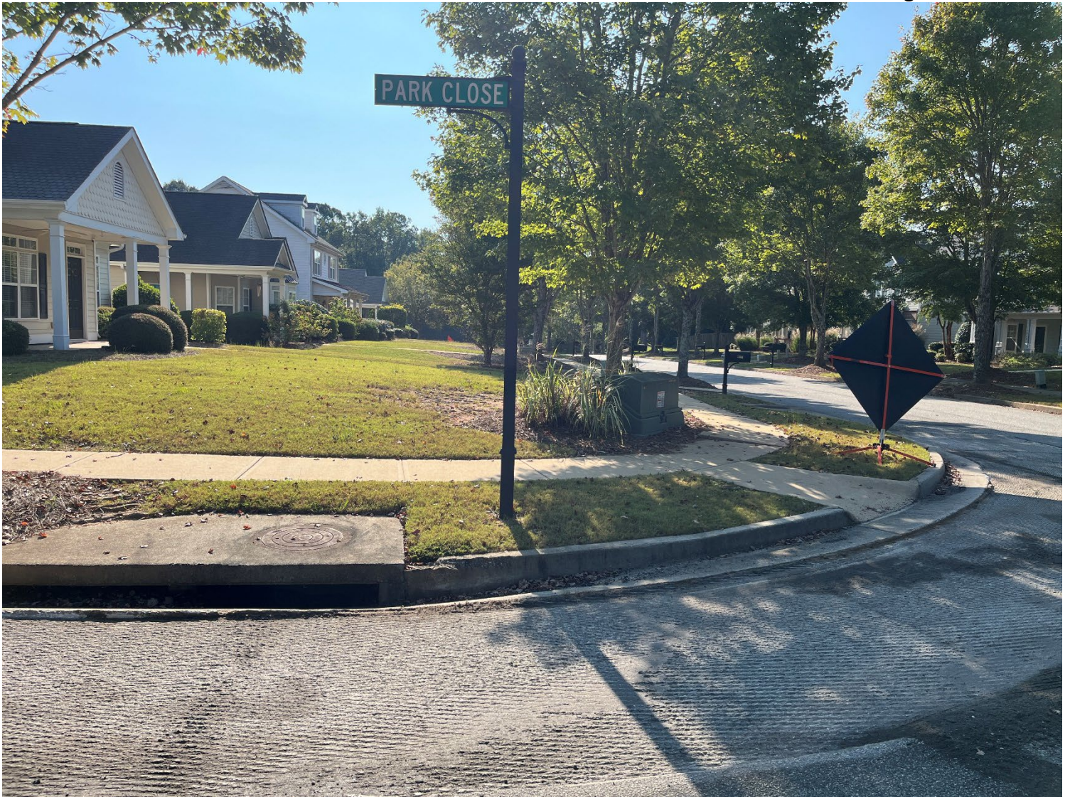
First Road Milled within The Lakes at Cedar Grove
