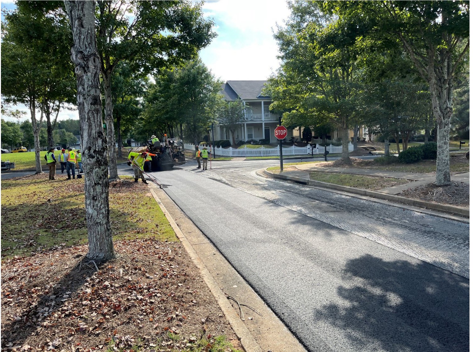
Complete paving operation on Park Close withing The Lakes at Cedar Grove
