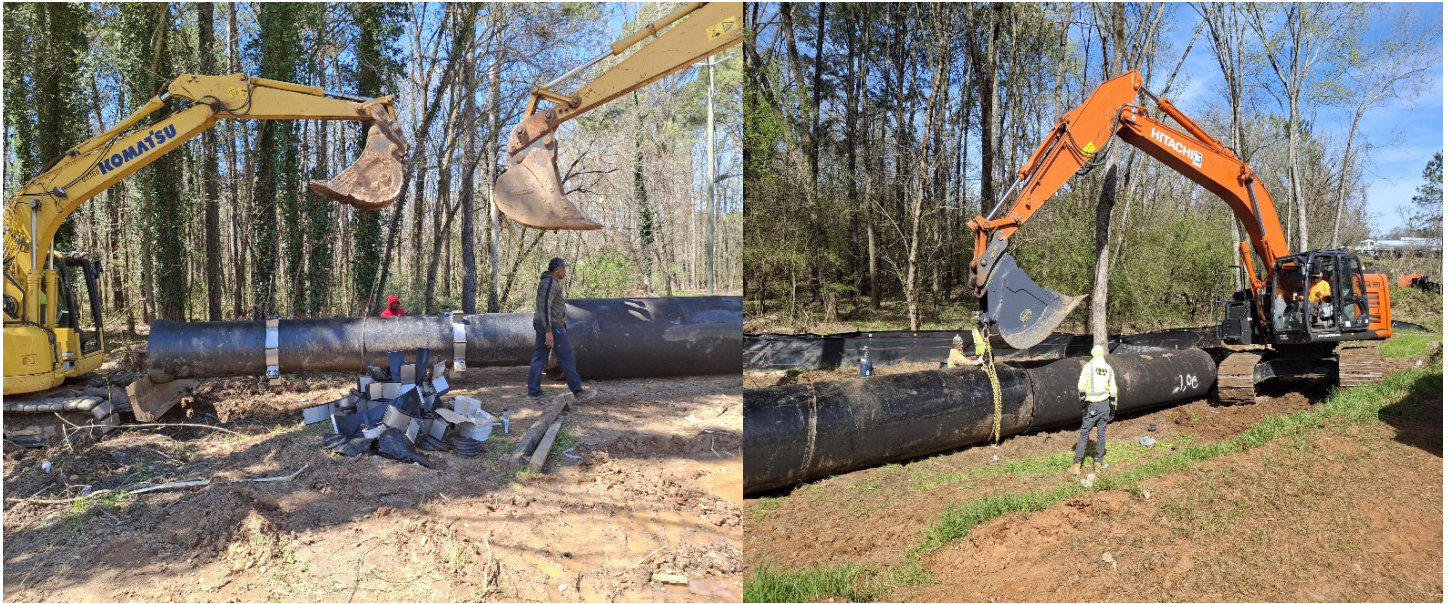
Bypass Casing Fabricate
