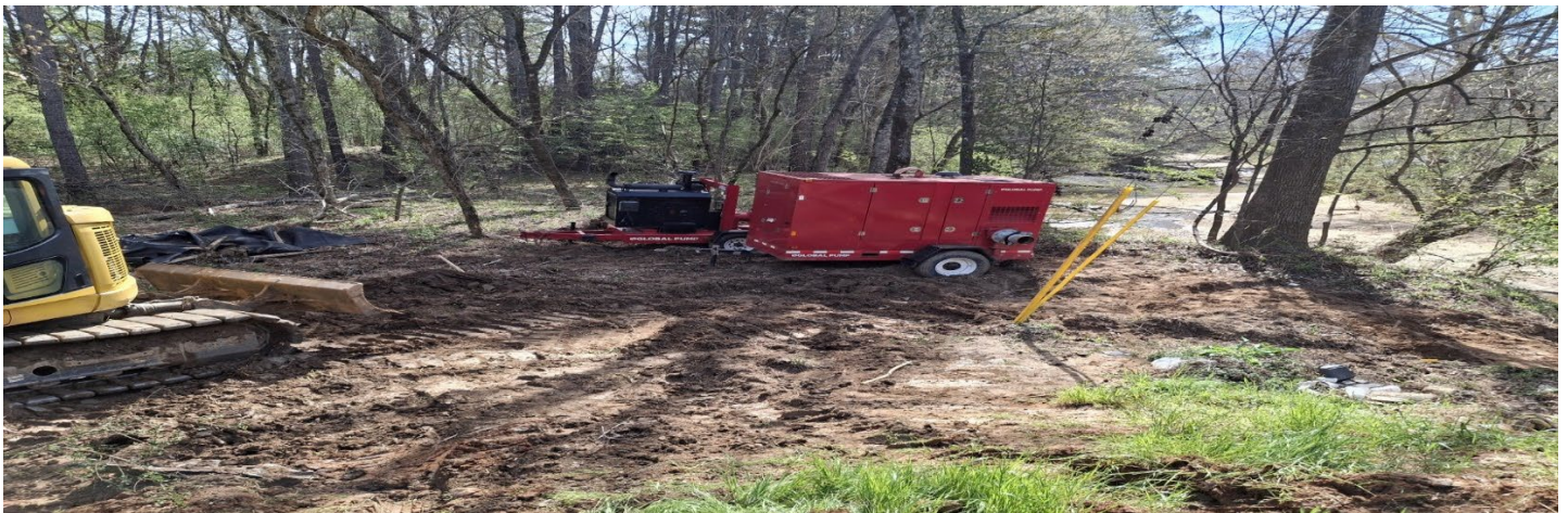
Pump set up to work
