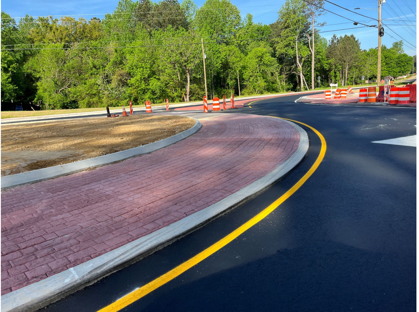
SD&C on-site grading center of roundabout along Butner Road and Union Road
