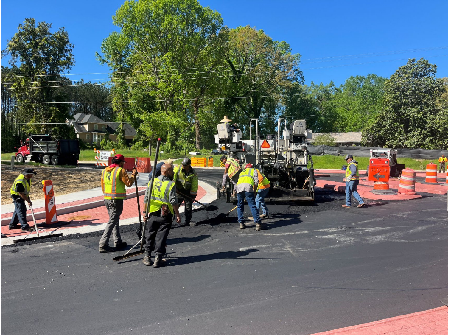
Triple "R" Paving on-site placing final lift of asphalt along Butner Road
