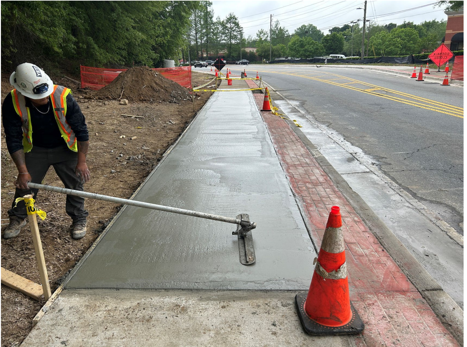
Sidewalk replacement by Primoris
