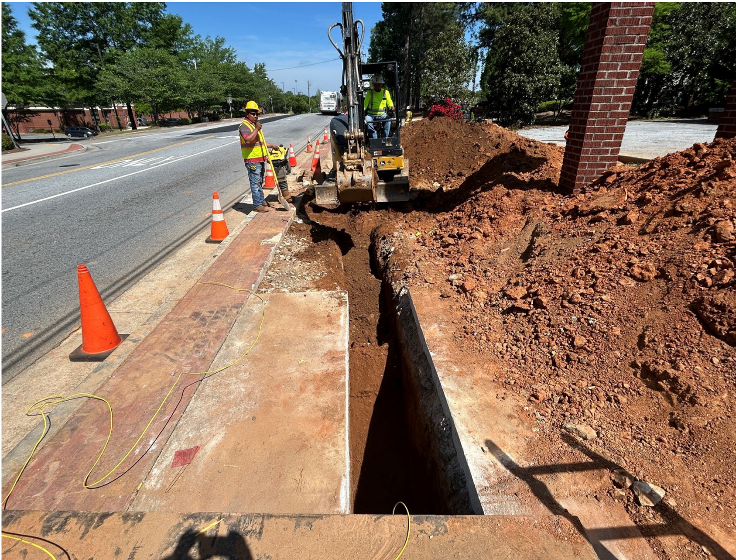
6in gas main tie-in
