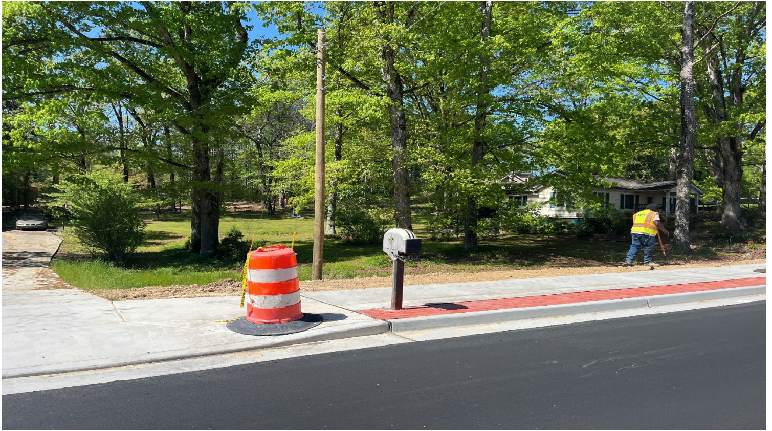
SD&C on-site grading and grassing shoulder along Butner Road and Union Road
