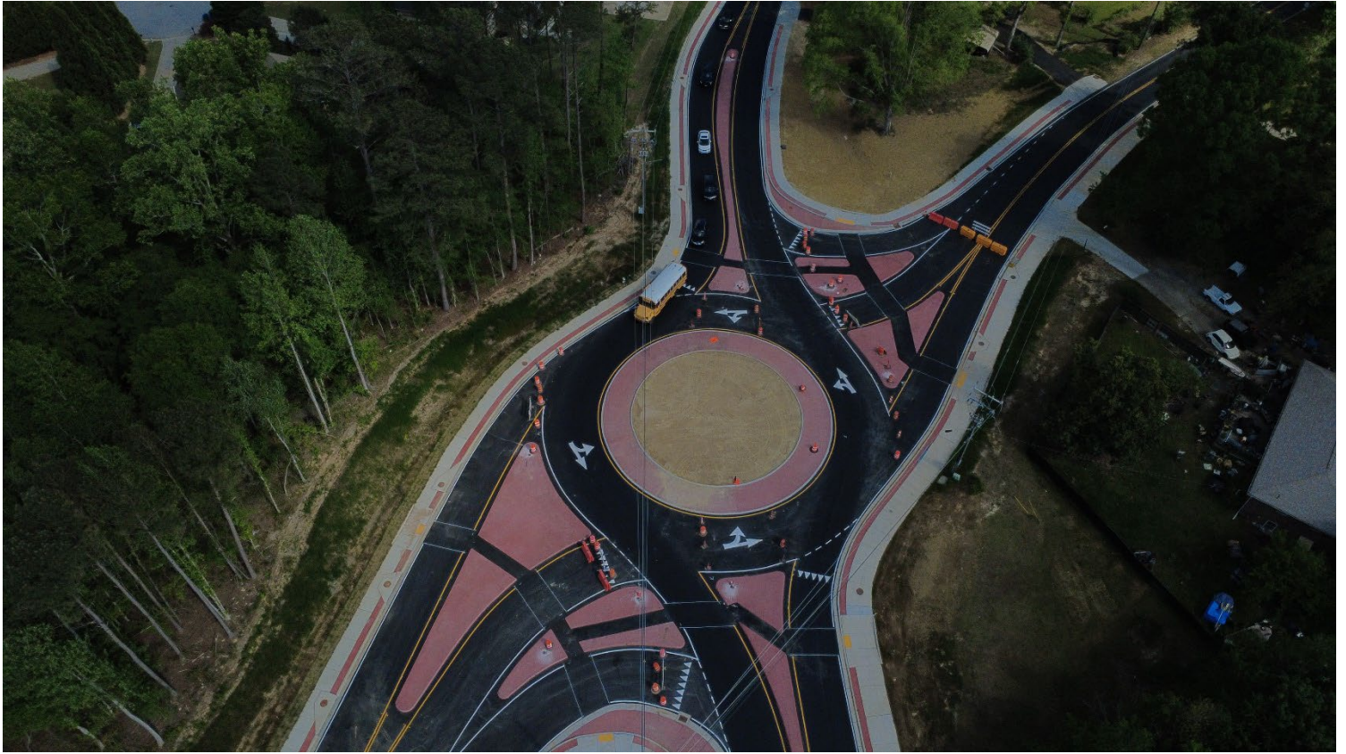
Jacobs on-site taking aerial photos Butner Road and Union Road Roundabout
