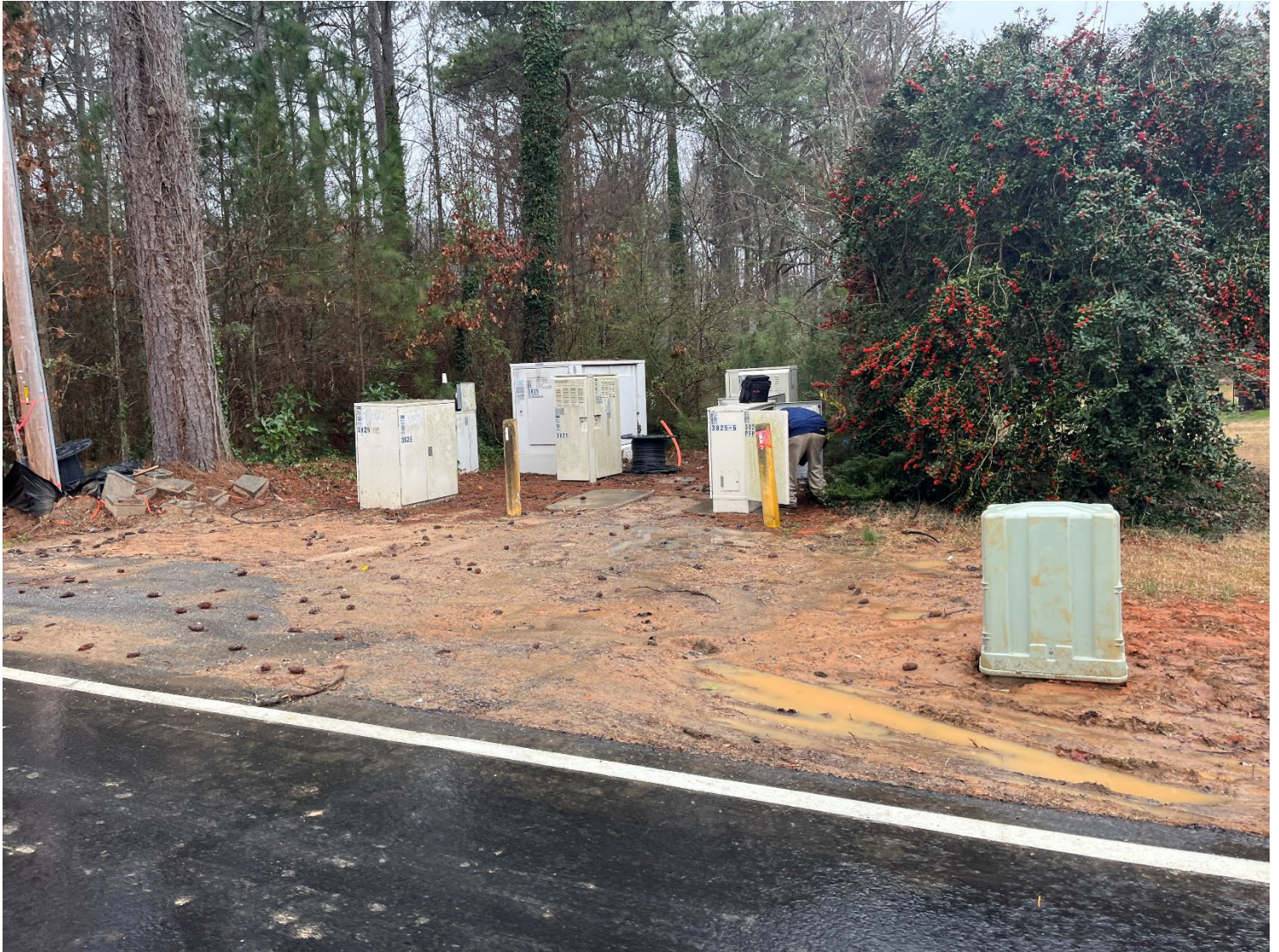
AT&T is working on corrective list items for underground wiring along Butner Road and Union Road
