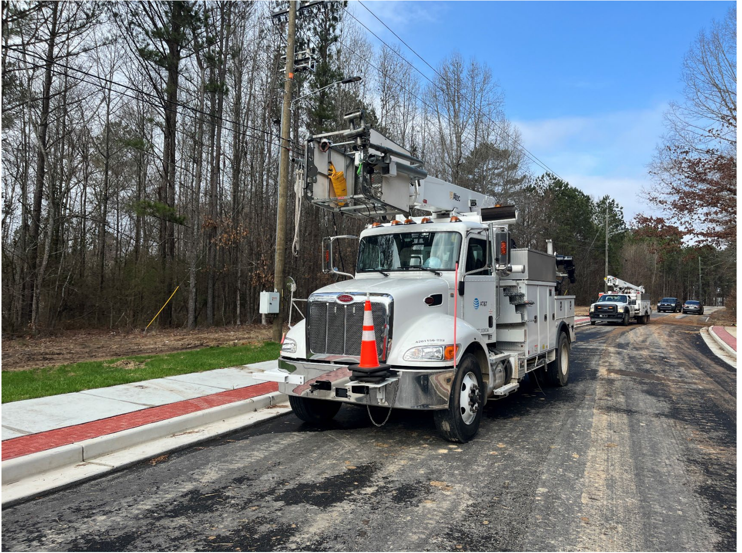
AT&T on-site removing aerial lines for cut over to new poles throughout project
