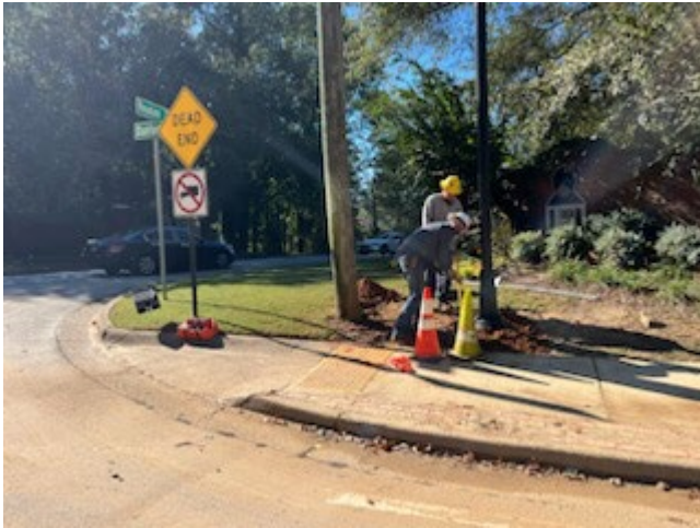
Ga Power Crews installing street lights
