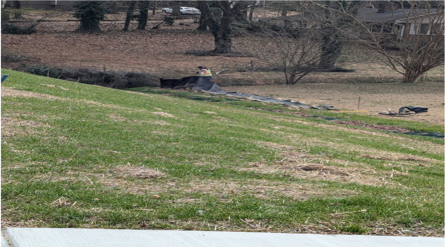
SD&C on-site removing silt fence from established vegetation areas (15+80 to 17+00) on Butner Road and Union Road
