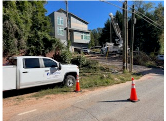
Ga Power Crews working on Power pole
