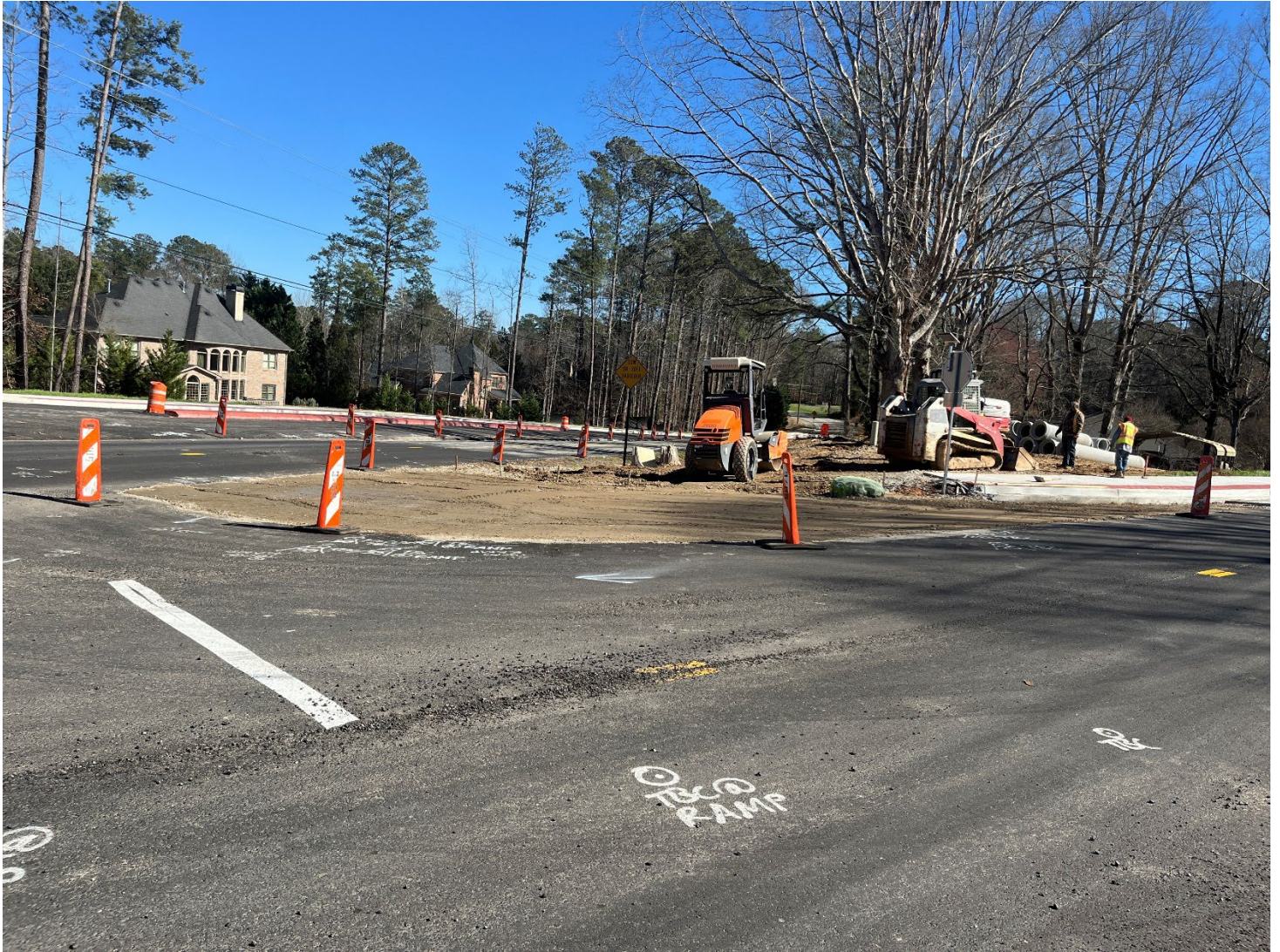
SD&C on-site grading radius for truck apron (40+00 to 18+00) and roadway along Butner Road and Union Road
