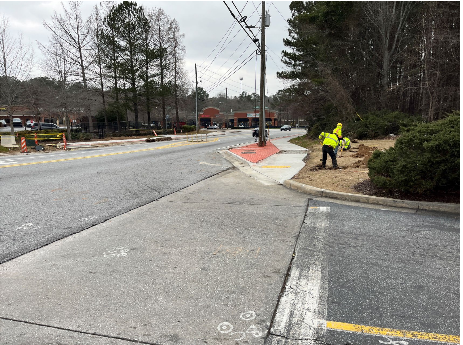
Potholing exiting gas line.
