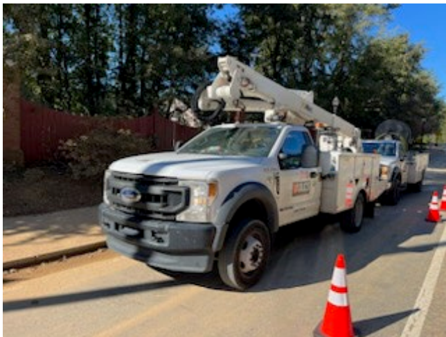
GA Power Crews working on Pole installation
