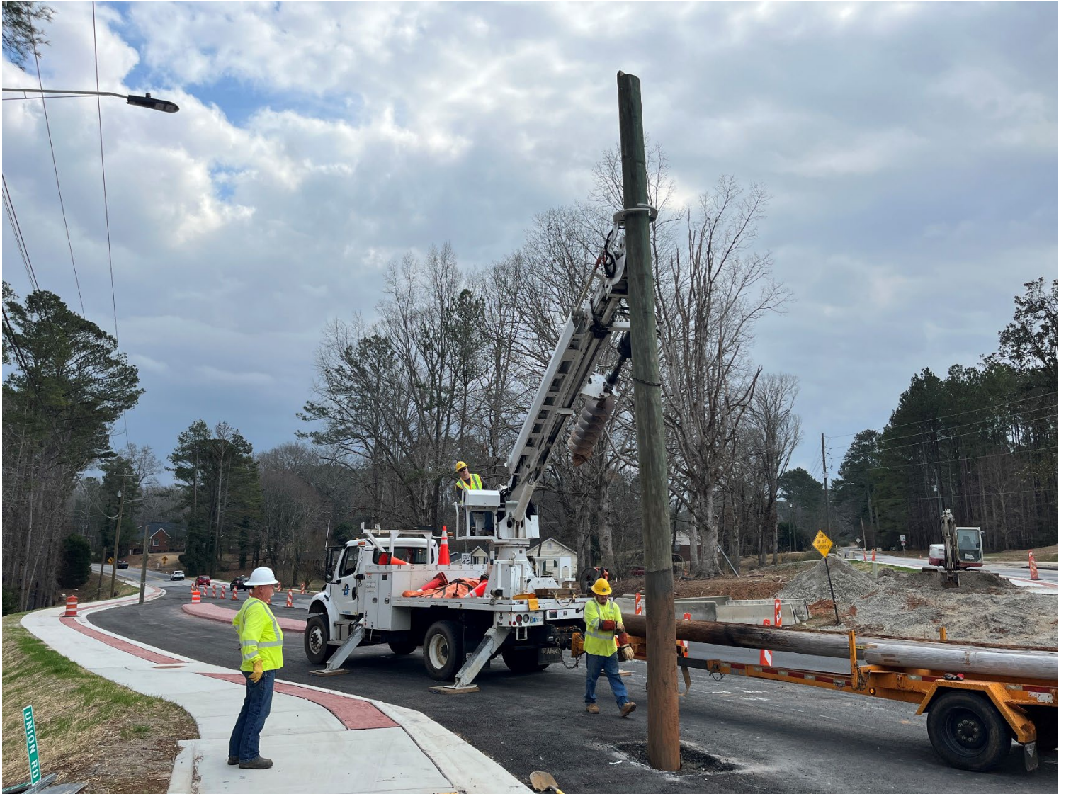
Greystone on site removing old AT&T poles from within the roadway
