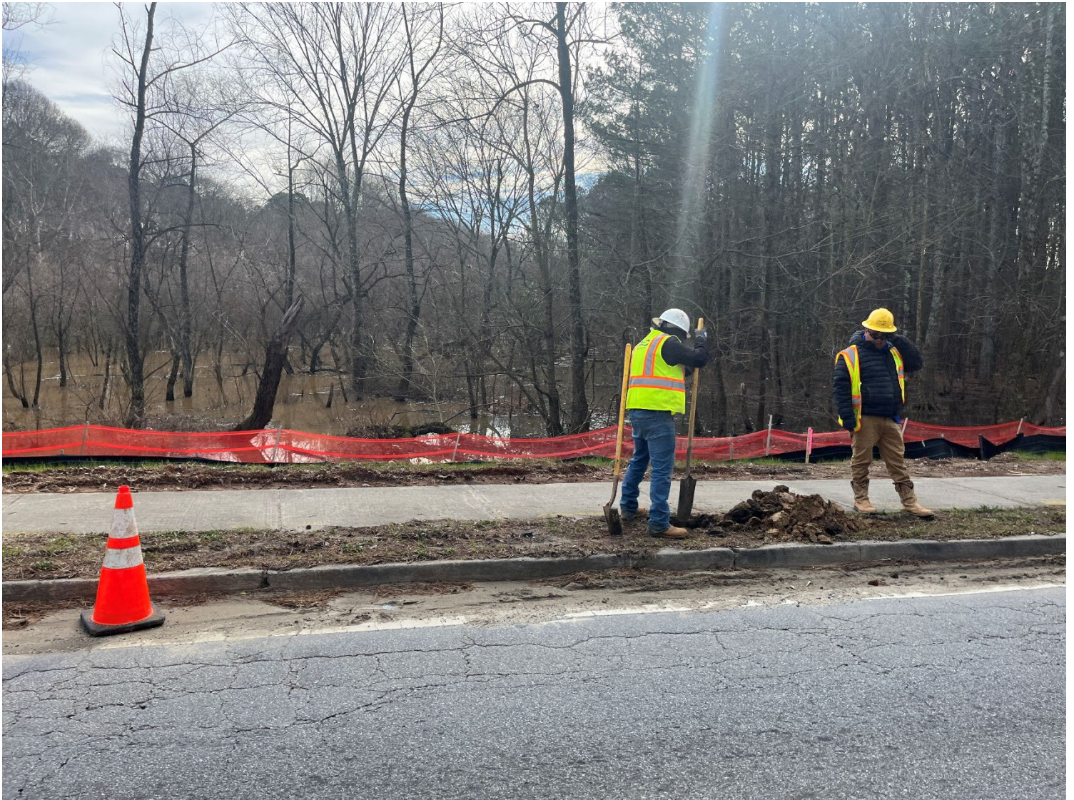
Locating existing gas line.
