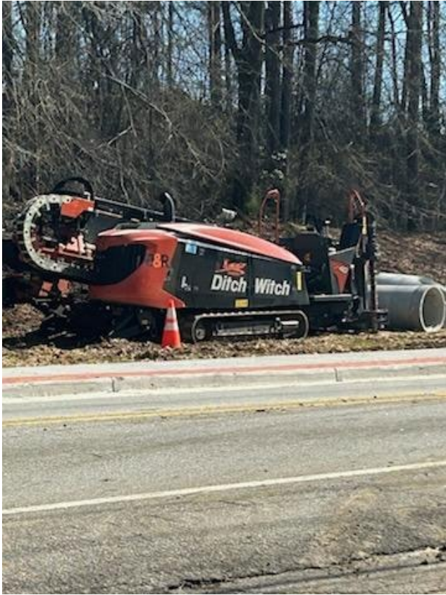
Installation of Gas Line
