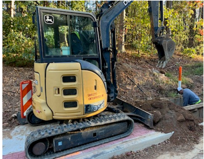
GA Power Crews working on Pole installation
