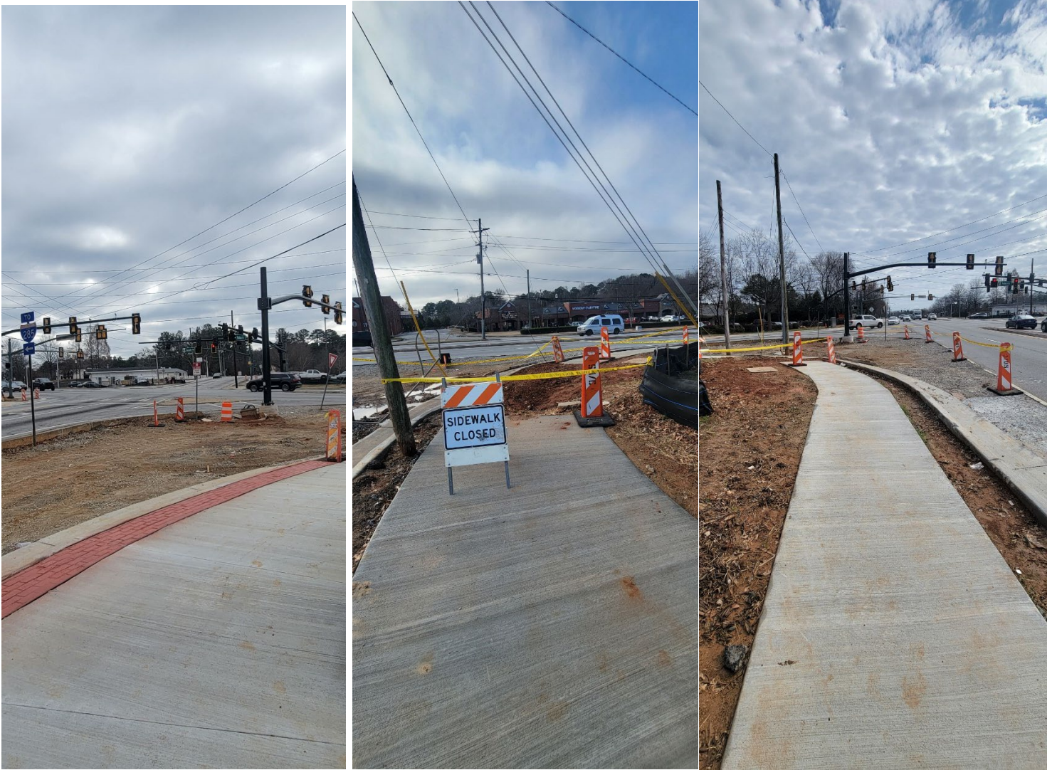
Locations awaiting gas line relocations
