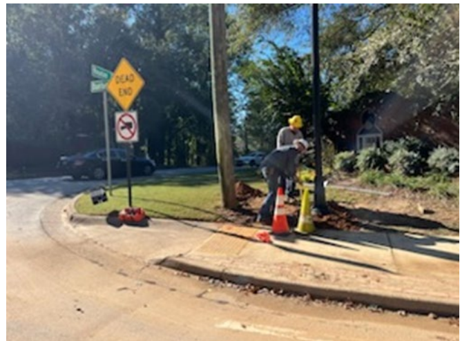
GA Power Crews installing Street Lights
