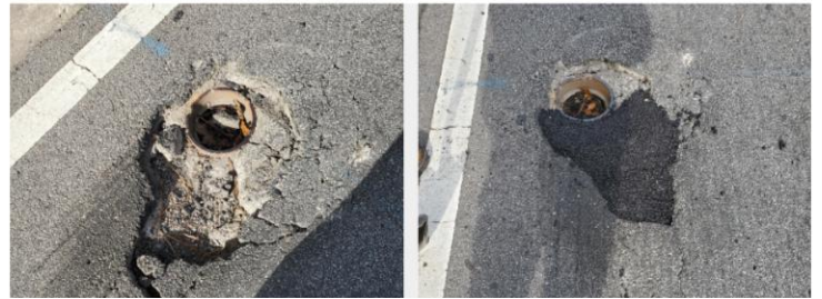
Pothole repair along New Hope Rd December 2020
