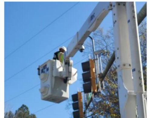
Work being performed at Danforth November 2020
