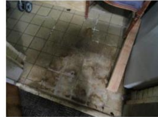
Damaged Quarry Tile Flooring
