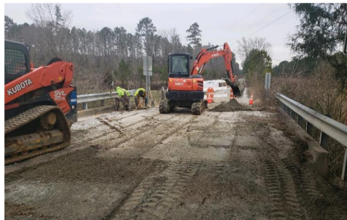
Repairs to sinkhole on bridge January 2021
