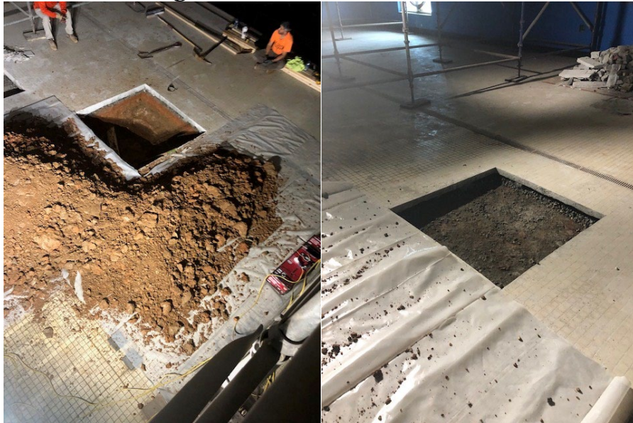
Footing Excavation for Slide at Pool
