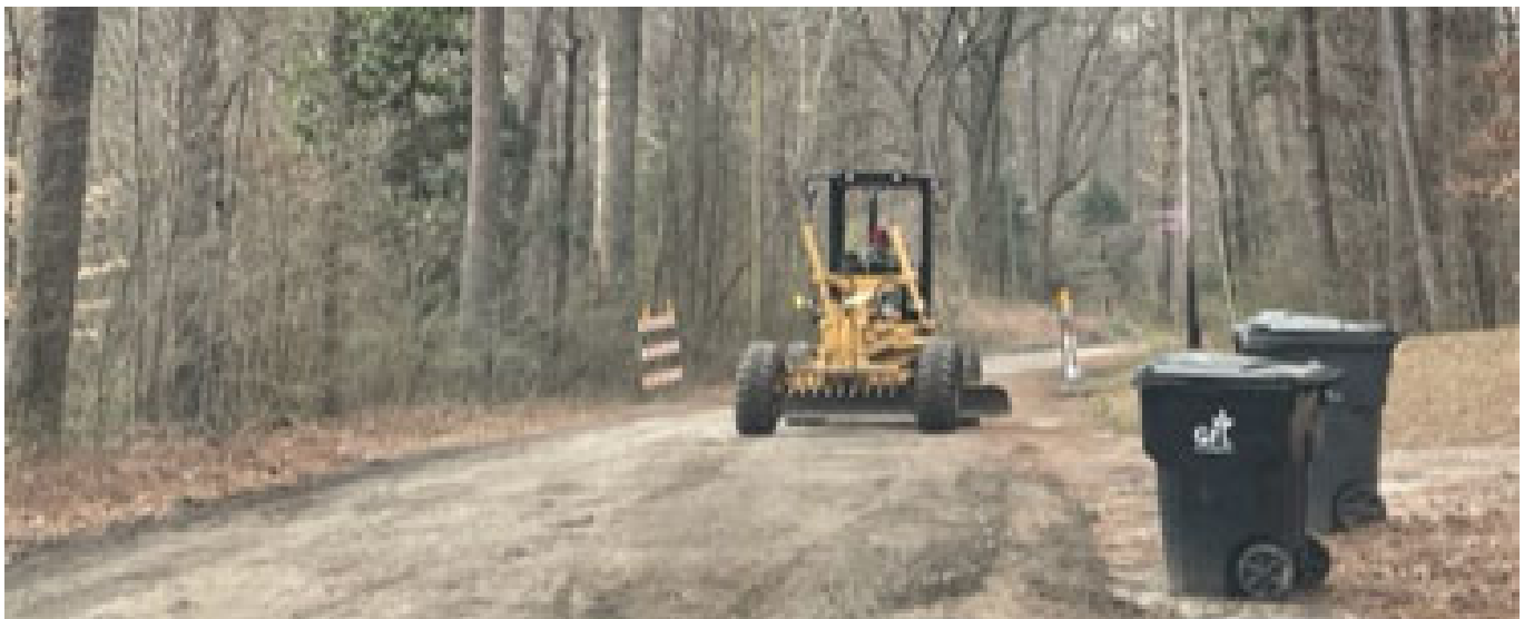
Gravel road maintenance on Jones Road
