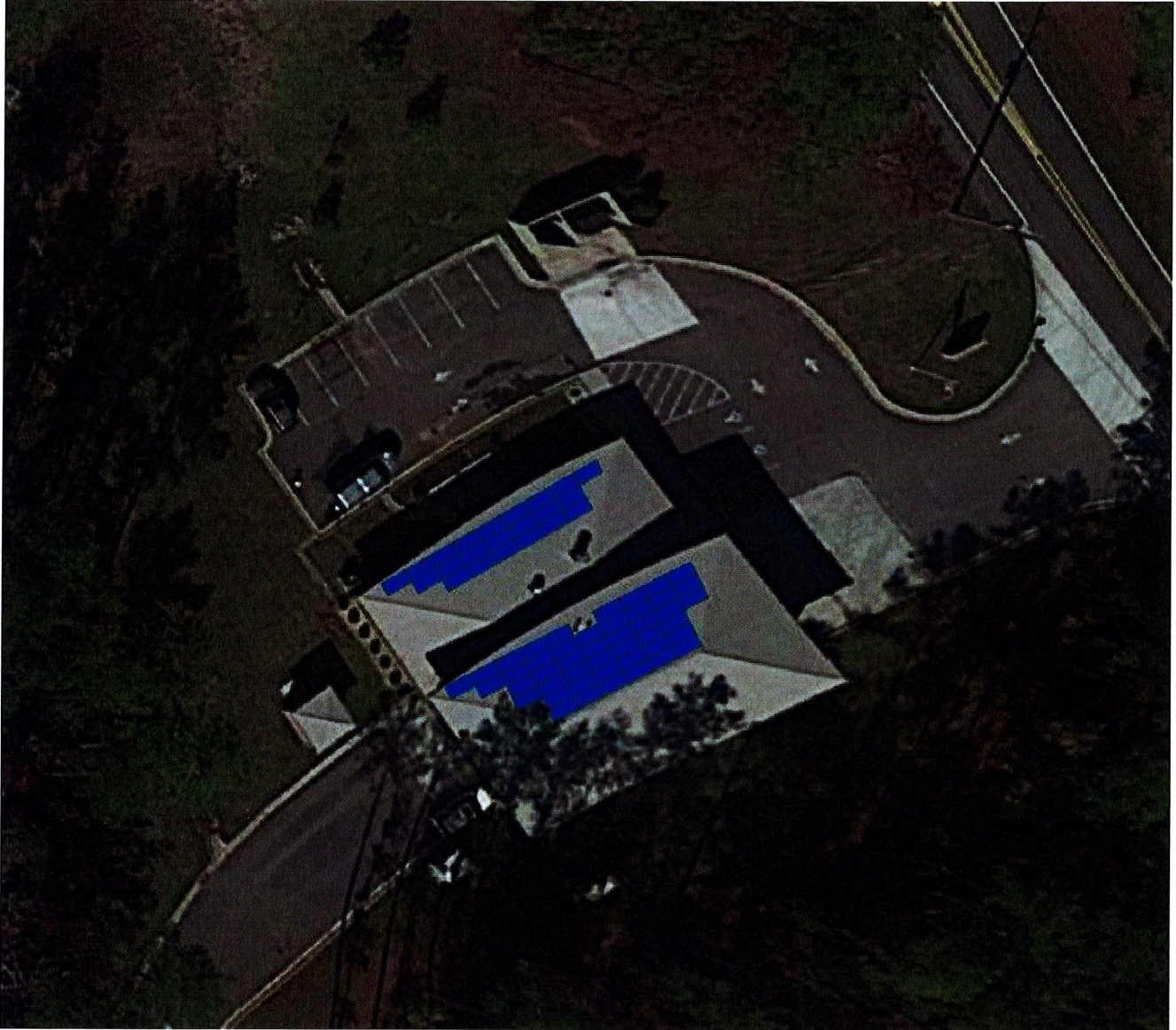
Figure 2: Solar roof-mounted system on north/northwest roof surfaces
