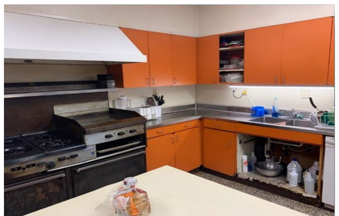
Previous Hood, Stove, Cabinets
