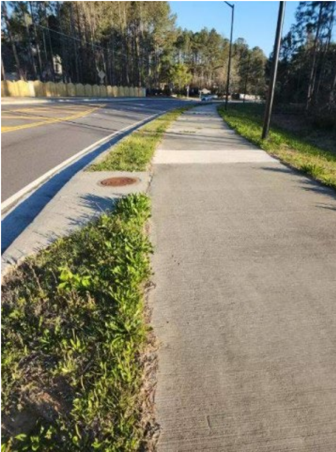
Campbellton Road - Before
