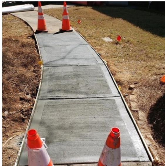
Sidewalk Repair at Waterlace Drive March 2021
