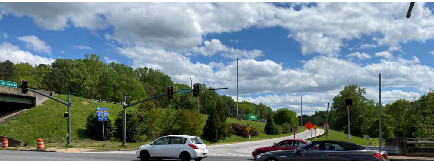
PHOTO 4: Overview – I285 Northeast On Ramp
