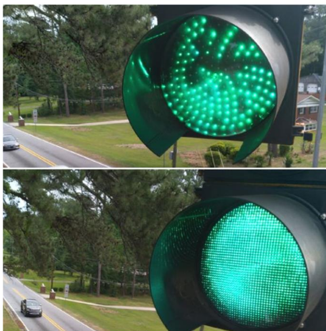
Before and After LED Light Replacement Flat Shoals Rd & Red Oak Rd
