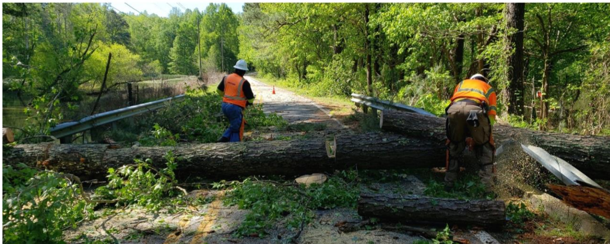
Public Works Crews Removing trees from Short Road.
