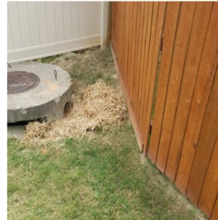
Repairs to Sinkhole at Flyaway Road May, 2021
