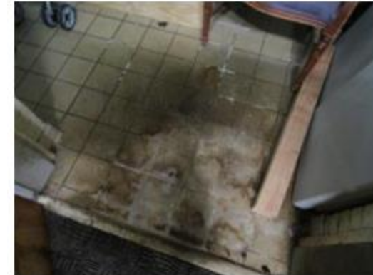
Damaged Quarry Tile Flooring
