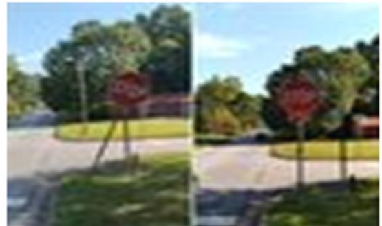
Down Stop Sign and Repairs at Valley Bend Rd & Kimberly Mill Rd. September 2021
