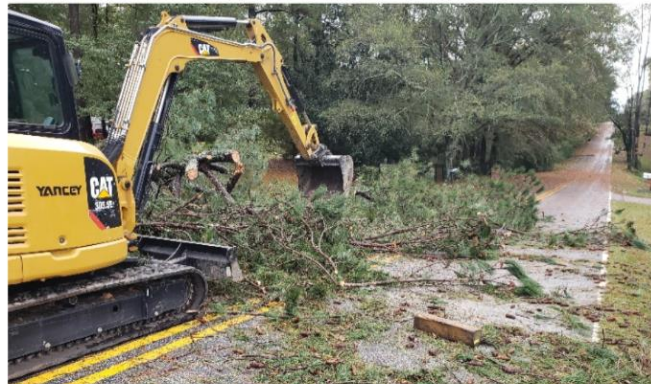
Crews remove trees & debris on Reynolds Rd October 2020
