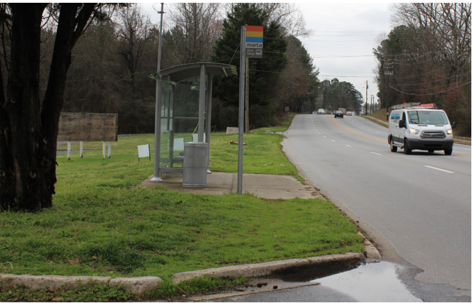
Figure 3-2: The only bus shelter on the corridor, with no sidewalk or curb cut present.
