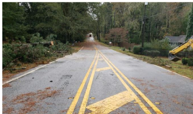
Reynolds Rd after crews removed trees from roadway. October 2020
