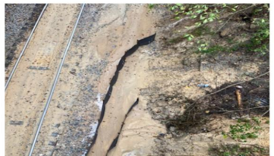
Silt fence installed to prevent mud from covering tracks. October 2020
