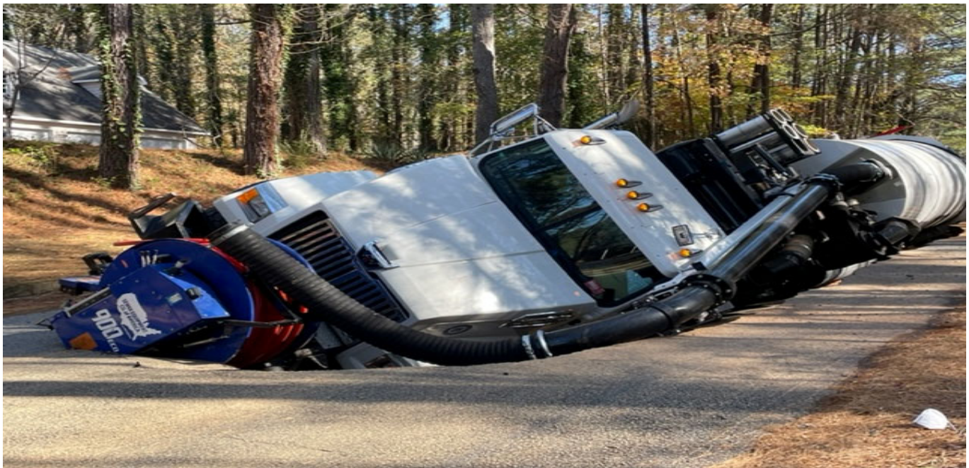
Orkney Lane road repairs underway due to sinkhole
