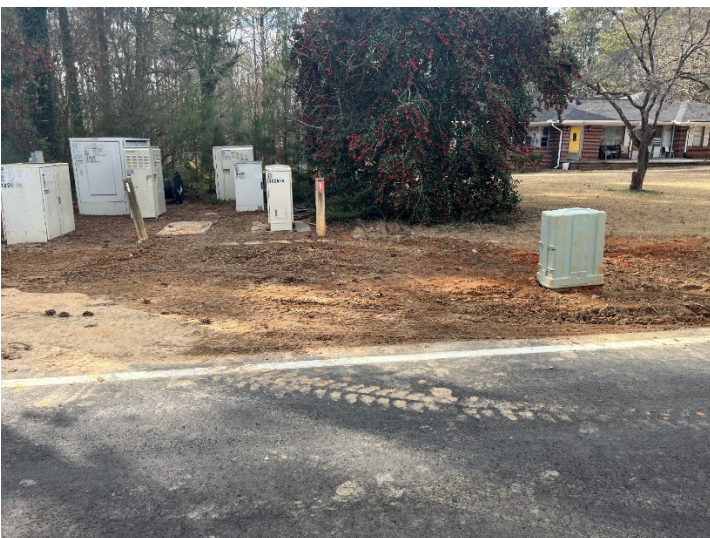
AT&T has completed underground wiring splice and backfill work
