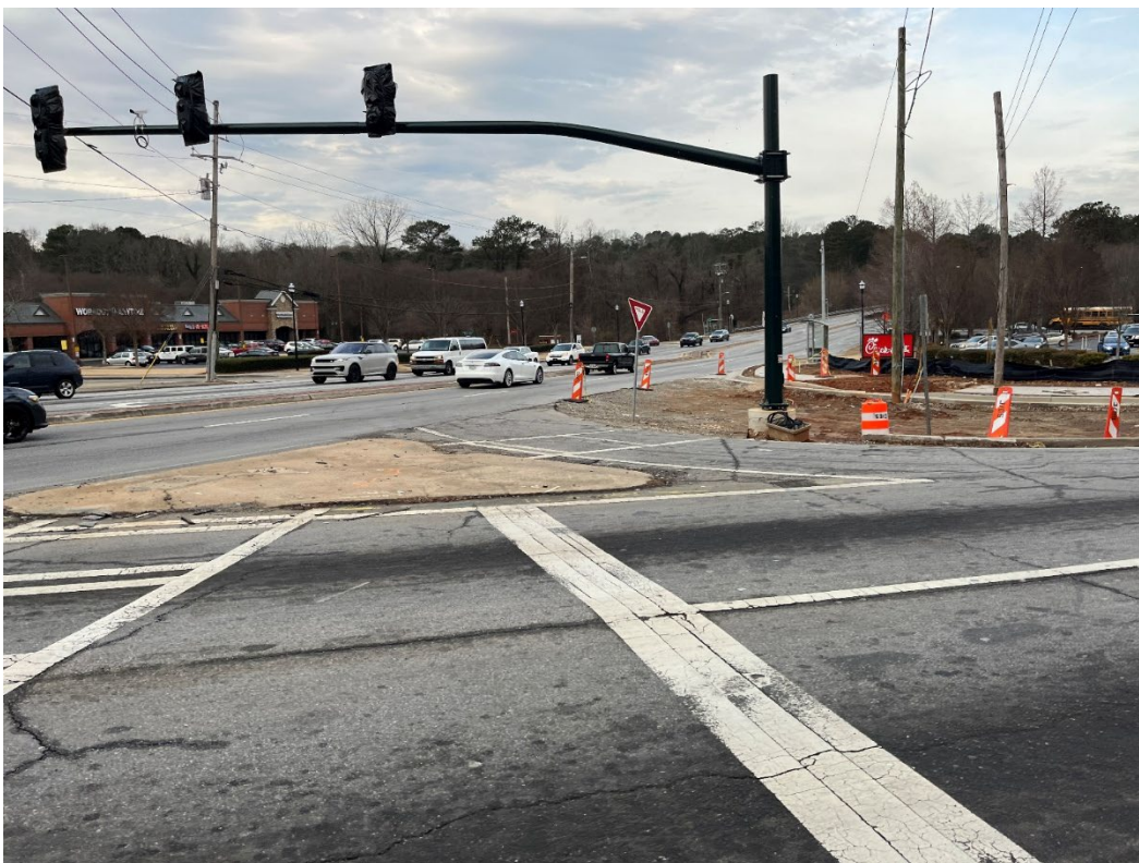
Reedwick on-site installing Traffic Signal Heads
