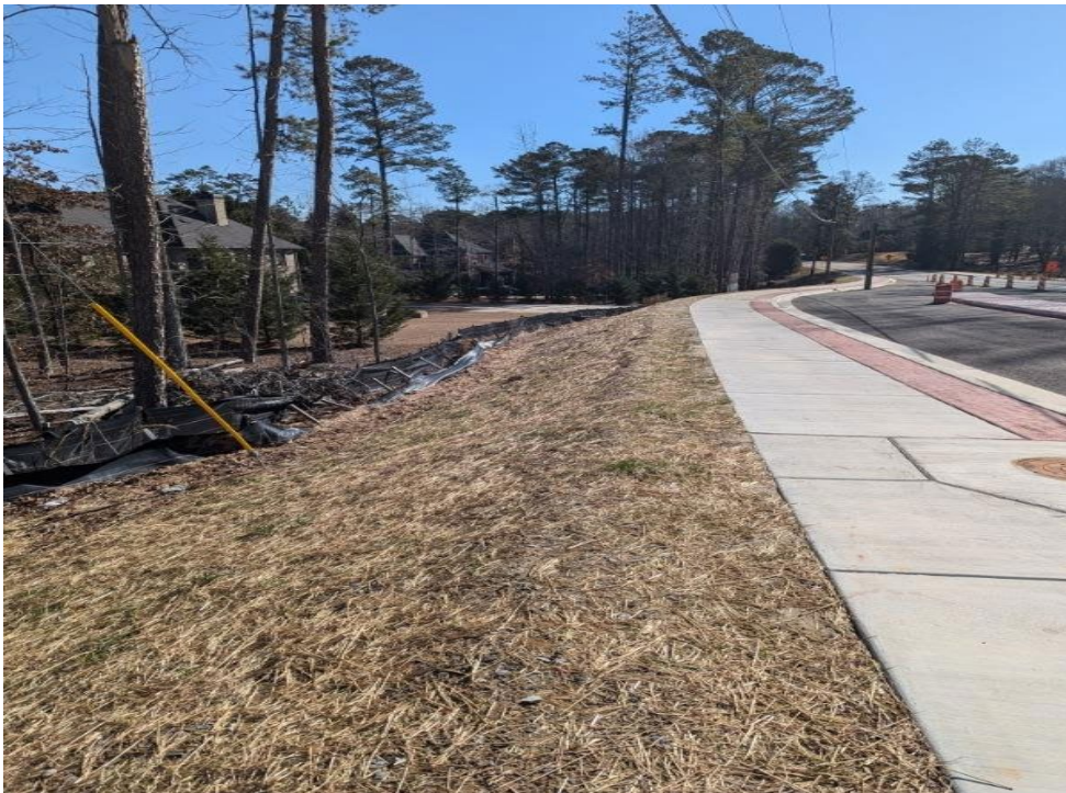
SD&C on-site placing permanent grass seed and mulching throughout project
