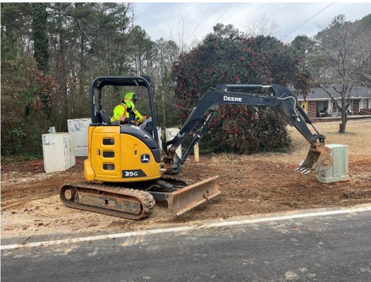
AT&T (ANSCO) on site backfilling underground wiring hole
