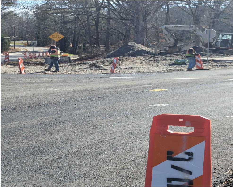
SD&C on-site evaluating possible New Traffic Pattern Layout on Butner Road and Union Road
