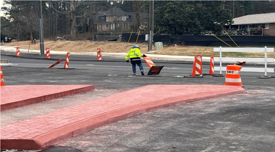
SD&C on-site addressing Erosion Control and Traffic Control items on Butner Road and Union Road
