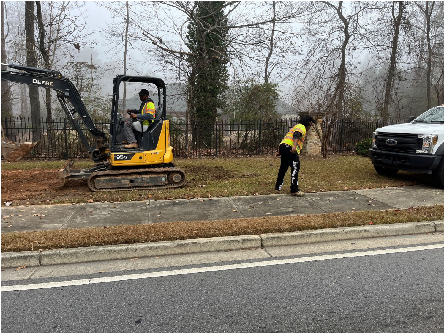
AT&T (ANSCO) on site backfilling underground wiring hole
