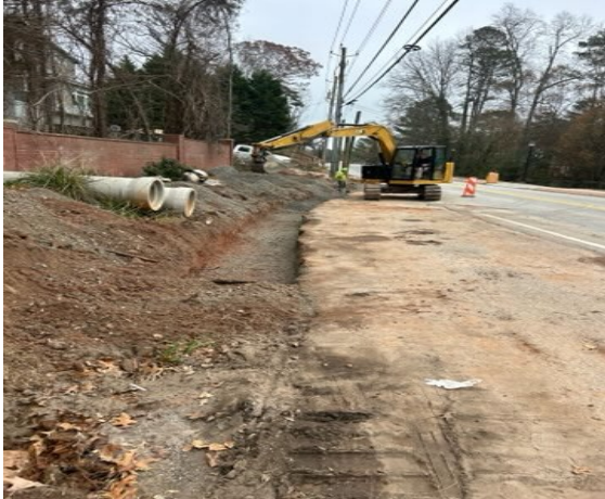
CMC grading for curb/gutter
