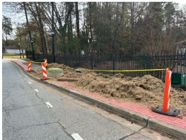
CMC excavating for drainage structure
