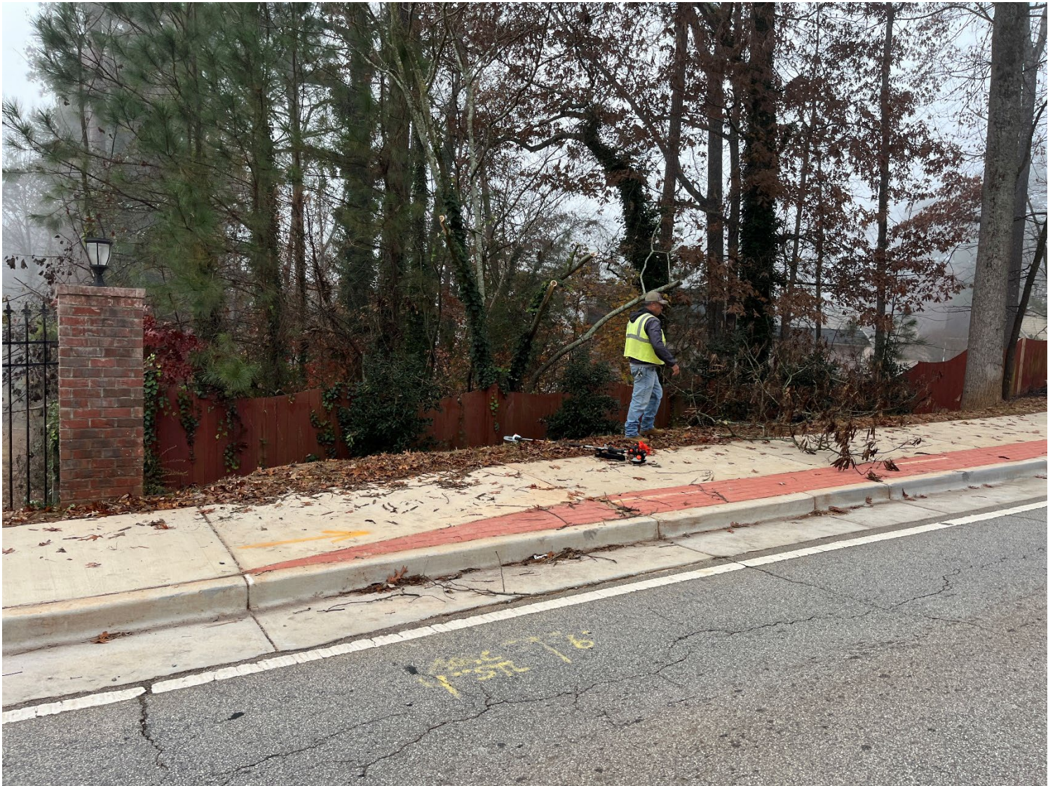
CMC on-site clearing within the right of way
