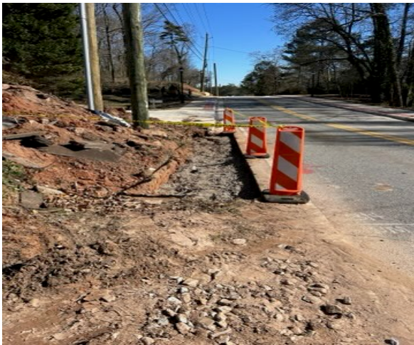
CMC placing G.A.B for curb/gutter
