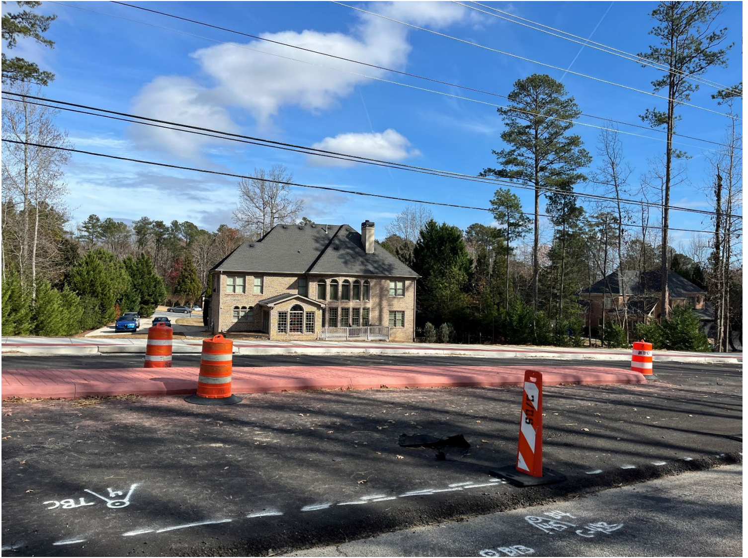
Color stamped concrete median
