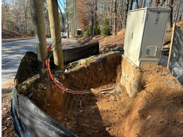
AT&T exposing underground wiring for box to be lowered
