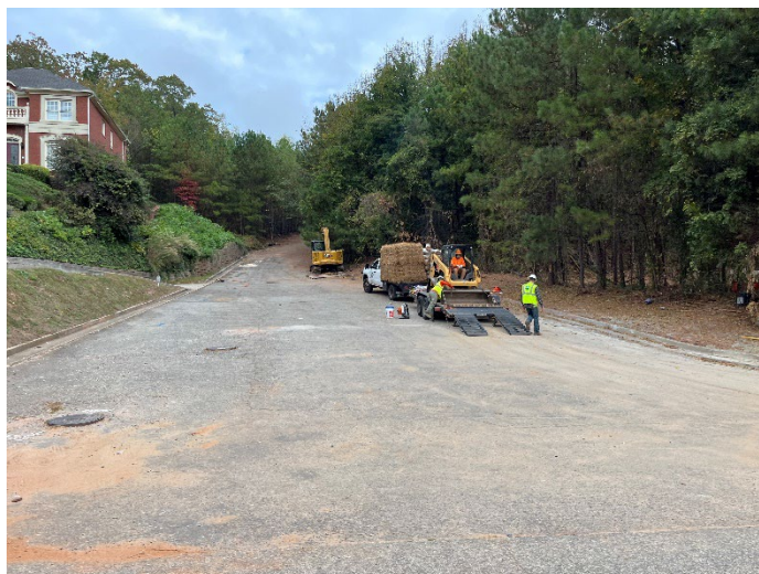
CMC on site mulching project 33
