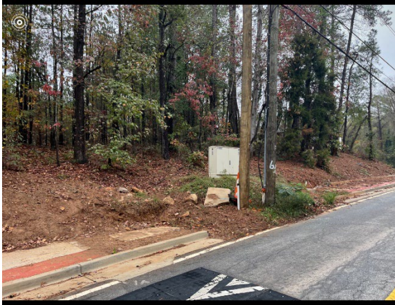
Power Poles and AT&T utility conflicts
