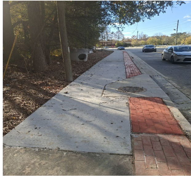
Sidewalk and Catch Base top C1
