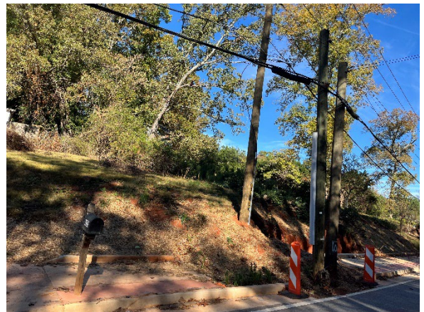
Power Poles are in conflict
