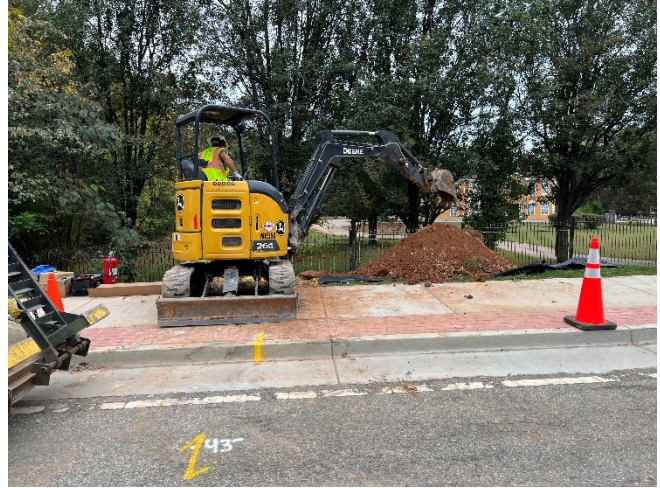
AGL (SEC) on site installing new gas line for newly constructed home
