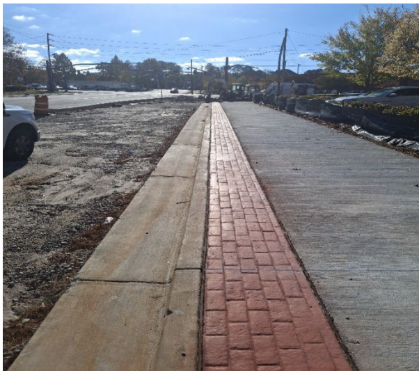
Sidewalk and Stamped concrete @ STA 148+00 – 149+00 LT
