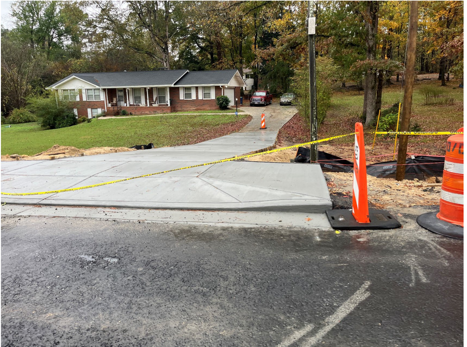
Driveway and Valley Gutter Completion
