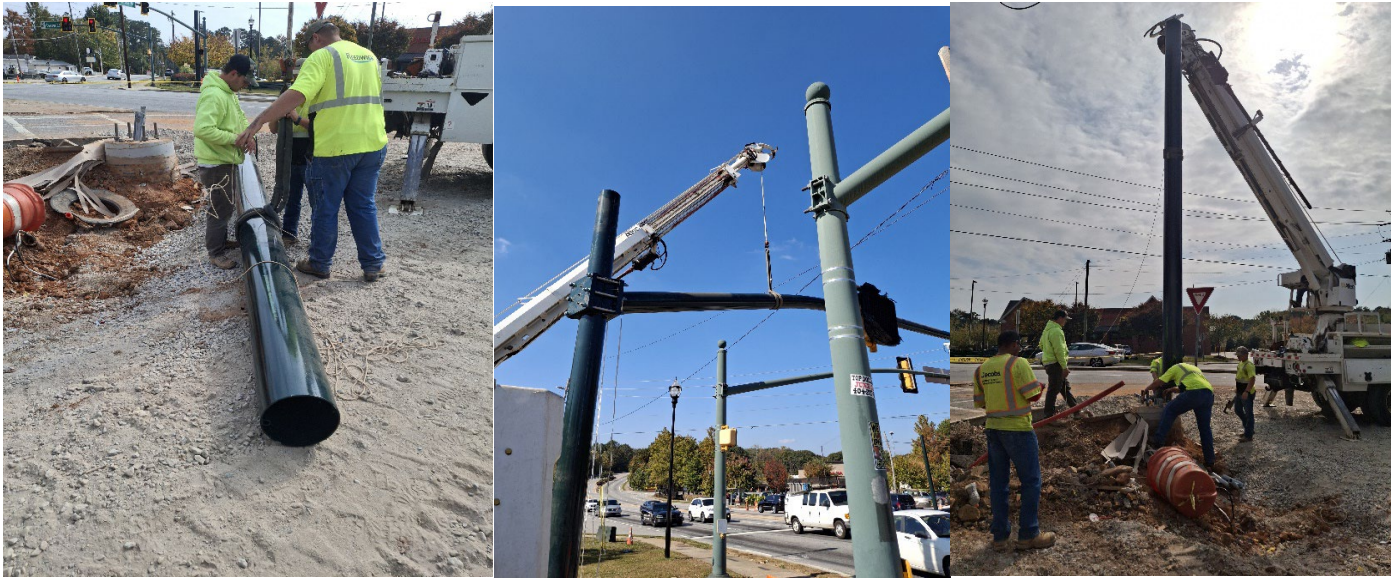
Strain Poles and Mast Arms installed @ corner of Fairburn Road and Cascade Road Intersection
