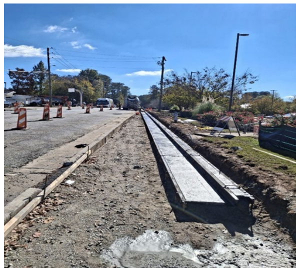
Curb & Gutter @ STA 144+50 – 146+50 LT
