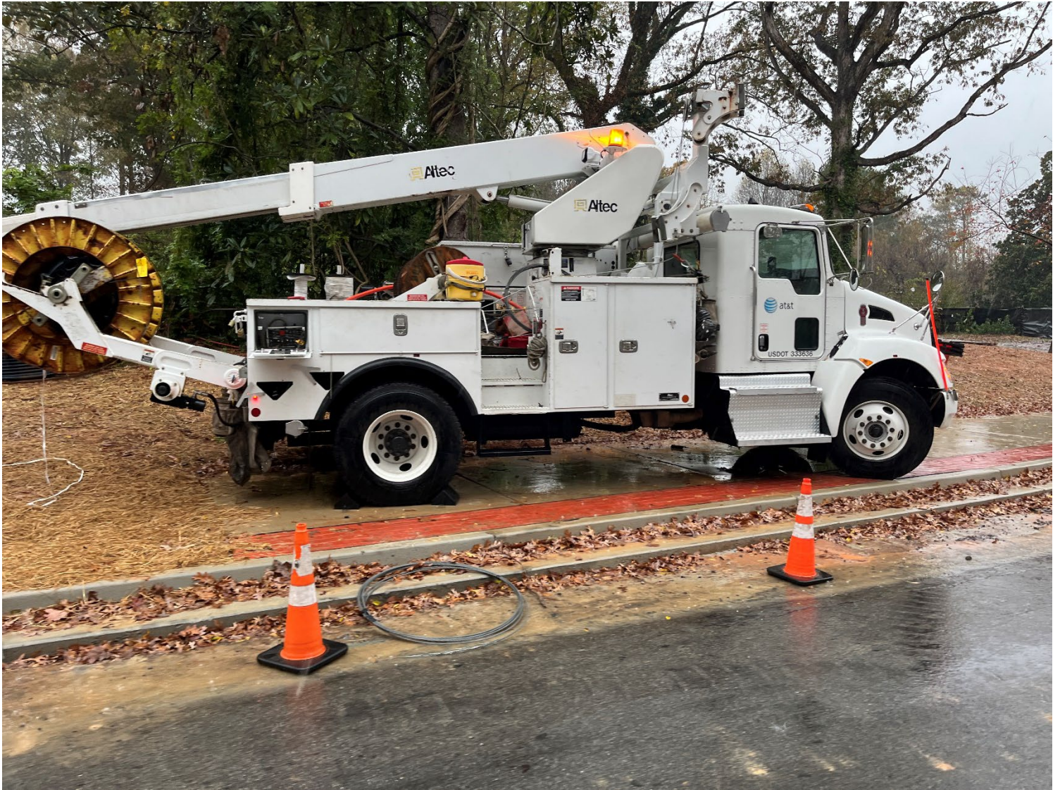
AT&T on site installing underground wiring
