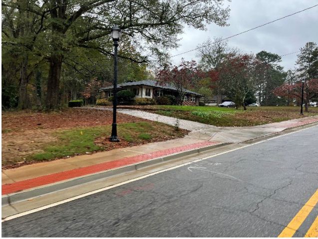
Pedestrian Street Lights on site
