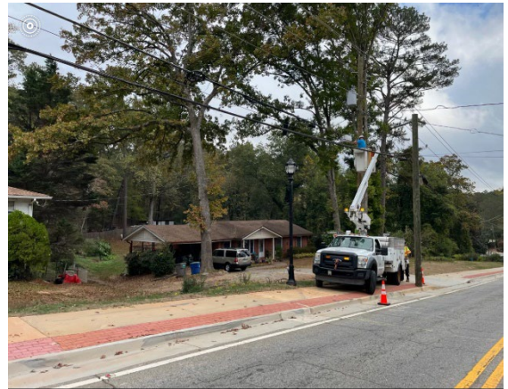
AT&T resolving one of many utilities conflicts
