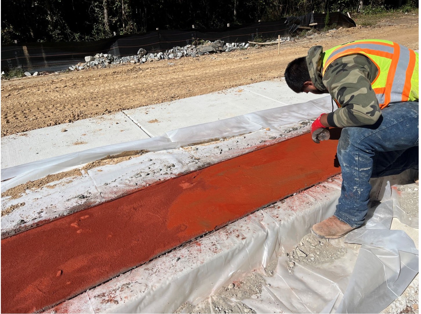
Placing color concrete for the beauty strip on Union Road and Butner Road
