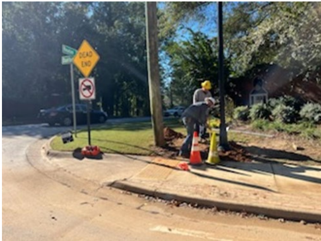
GA Power Crews installing Street Lights
