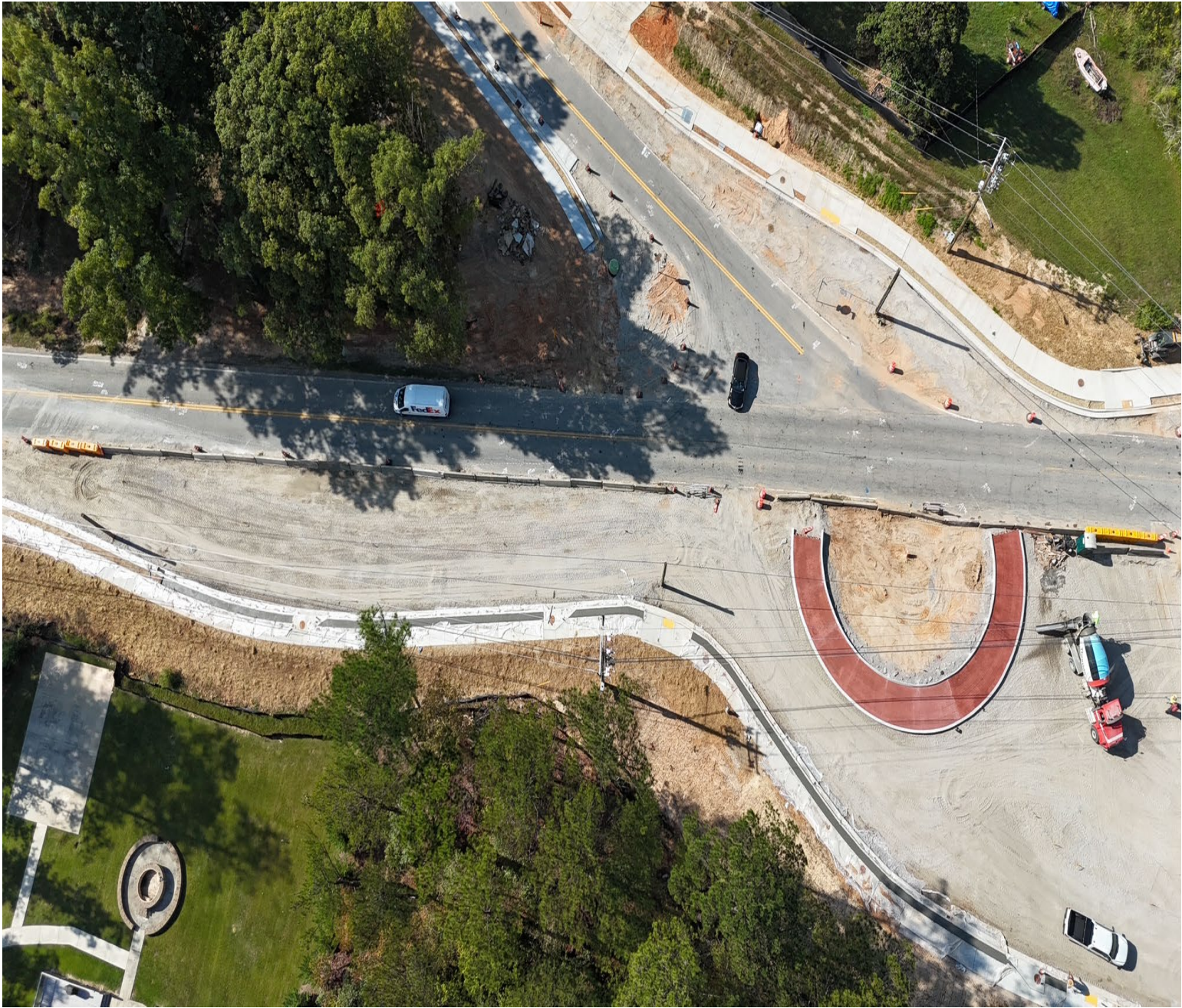
Aerial photo of work done in the month of October
