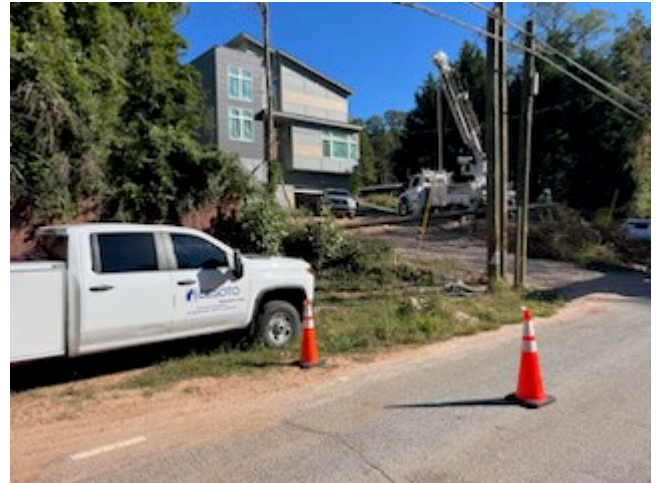
Ga Power Crews working on Power pole
