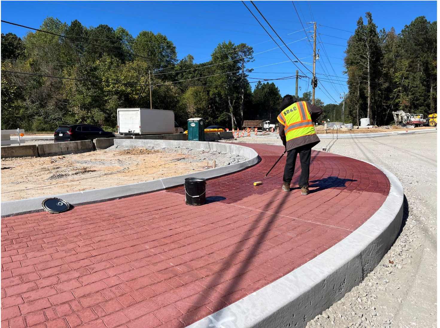
Applying sealer to the truck apron to preserve the color of roundabout on Union Road and Butner Road
