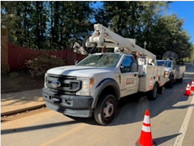
GA Power Crews working on Pole installation
