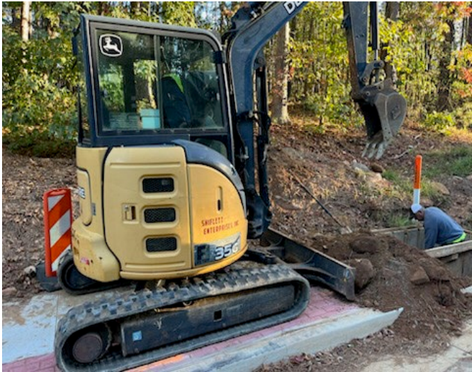
GA Power Crews working on Pole installation
