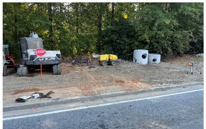
Projecting area for demo, curb/gutter and sidewalk
