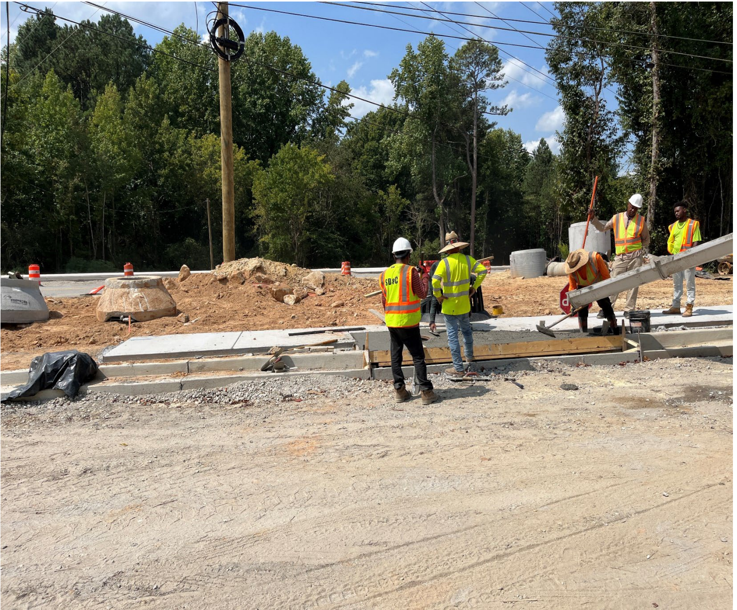
COMPLETED CATCH BASIN AT A 13
