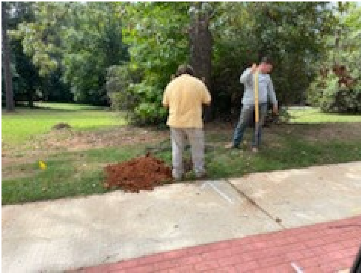
GA Power installing Street Lights
