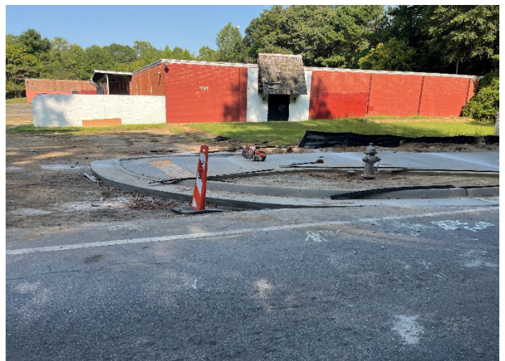
Curb/gutter, sidewalk and Ramp at station 155+50
