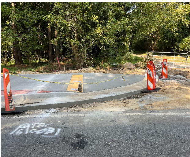
Curb/gutter, sidewalk and Ramp at station 158+85.
