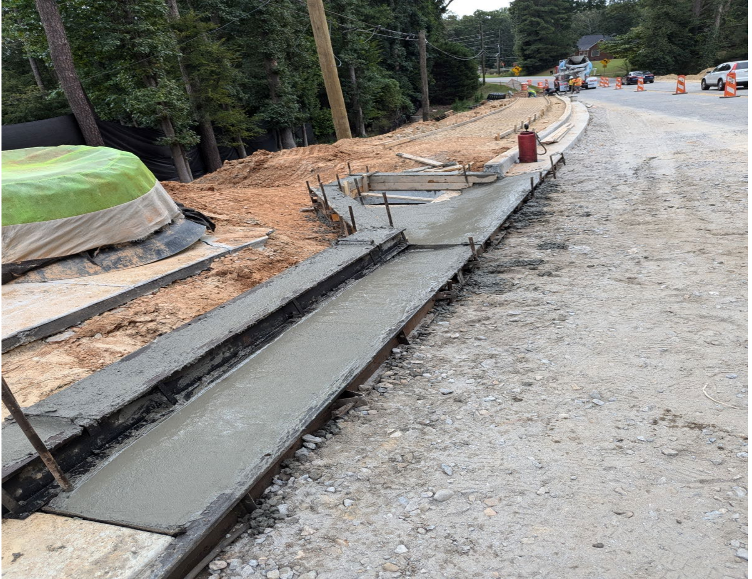
CURB & GUTTER AND SIDEWALK CONTINUE AT THE SOUTHERN SIDE.
