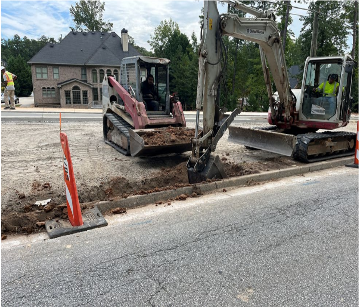
DEMOLISHING EXISTING CURB & GUTTER BETWEEN STATION 20+00 AND 26+00
