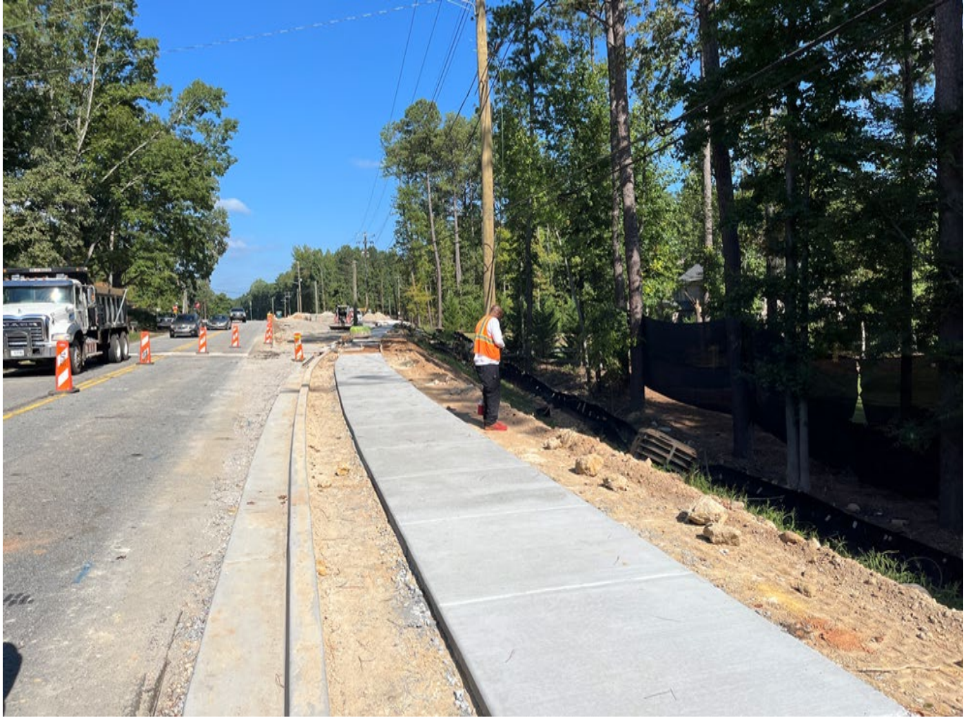
COMPLETED SIDEWALK FROM STATION 22+00 TO 26+00.
