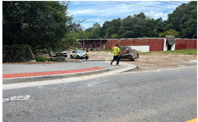
Curb/gutter, sidewalk and Ramp at Station 154+50
