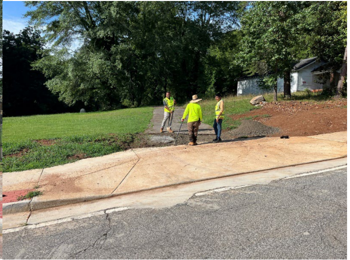
CMC grading for placement of asphalt for driveways
