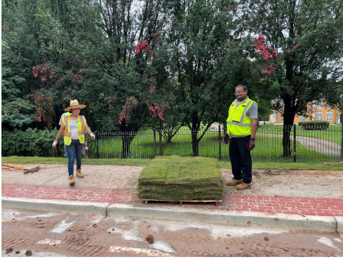
CMC on-site placing sod
